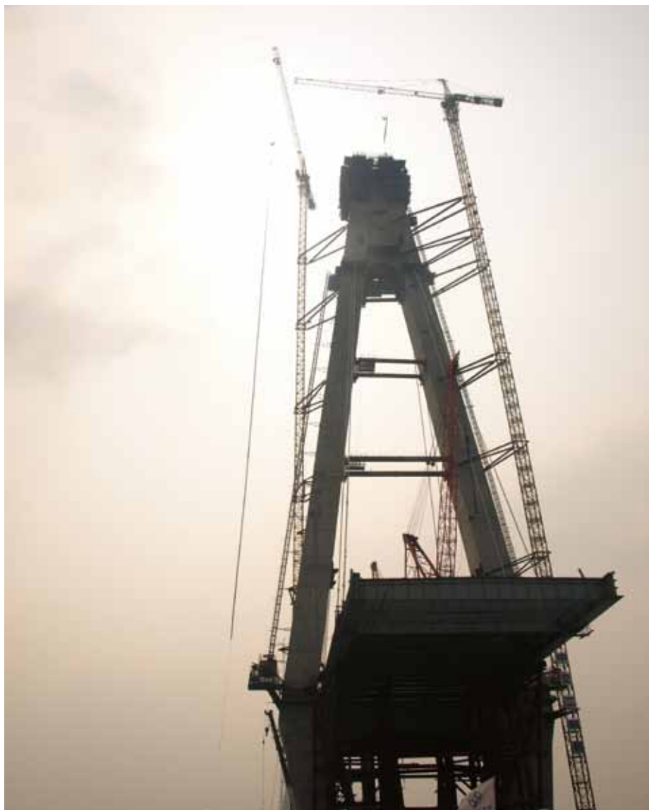
Erqi Yangtze River Bridge
