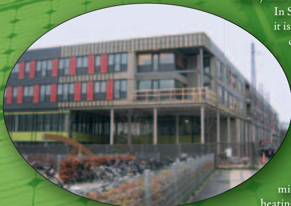
Elderly Centre Langgadehus finished March 2011.
