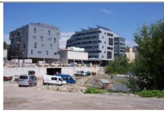
View of the buildings H and J with installed collectors
