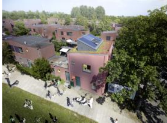
0-energy renovation from 2009 in Albertslund in Denmark with Solar Prism with PV mounted on the flat roof.
