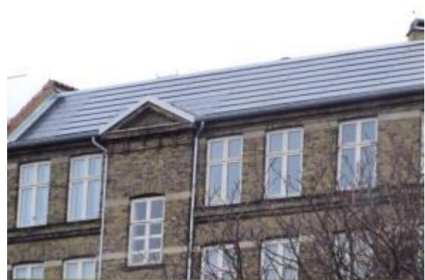
BIPV solution for "Søpassagen" housing project in Copenhagen
