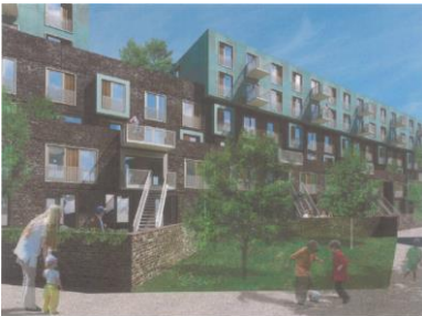
KAB low energy Class1 housing project at Carl Jacobsens Vej in Valby.
