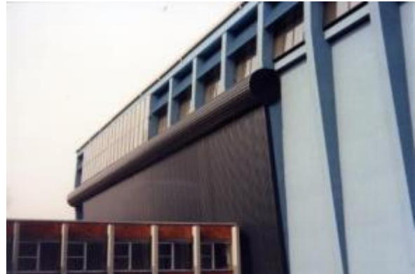
Solar research building renovated with Canadian Solar Wall preheating ventilation air
