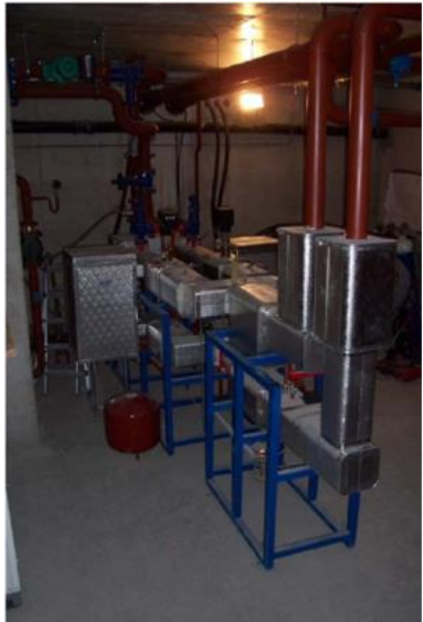
Solar station for 2000 m 2 collector area (left), District heating transfer station 1,5 MW (right)
