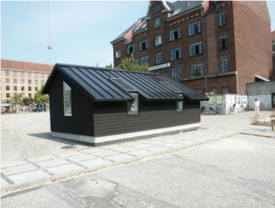
Development of zero energy test house in Denmark in 2003, which was exhibited in Valby.
