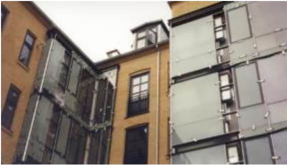
Urban renewal in the Hedebygade area in Copenhagen, with an example of a combined solar wall/ integrated heat recovery ventilation system operated by PV modules.
