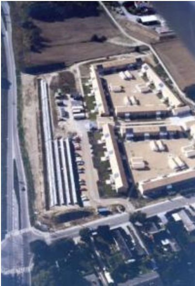
Solar plant with seasonal storage and heat pump in Herlev near Copenhagen
