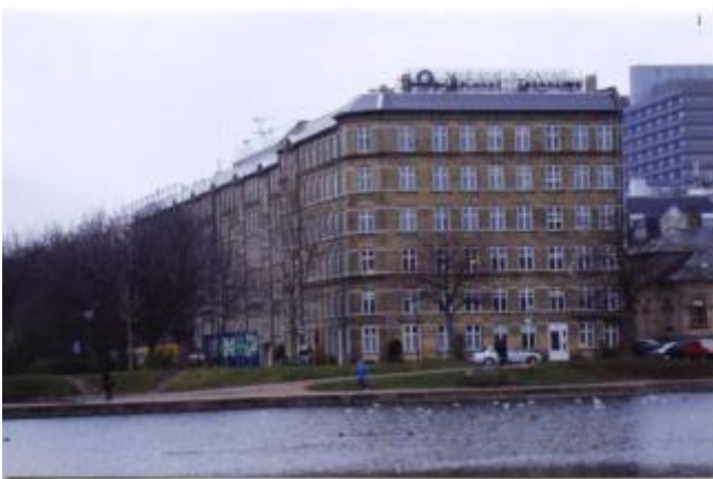
At the "Søpassagen" shared housing project existing shale roofs were changed to PV in a very nice way. Actually very few people notice that this is a PV roof.
