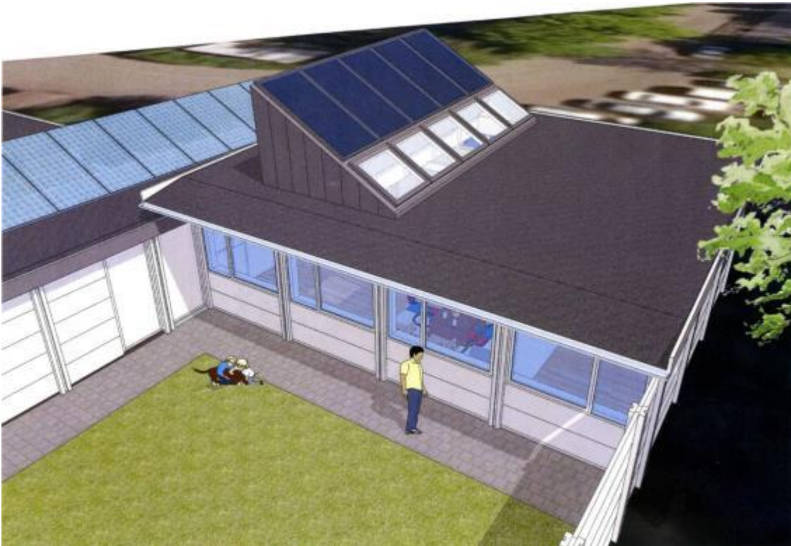
Example of housing area with courtyard houses renovated with solar energy combined heat and power (PV + Solar thermal in relation 1 : 1)
