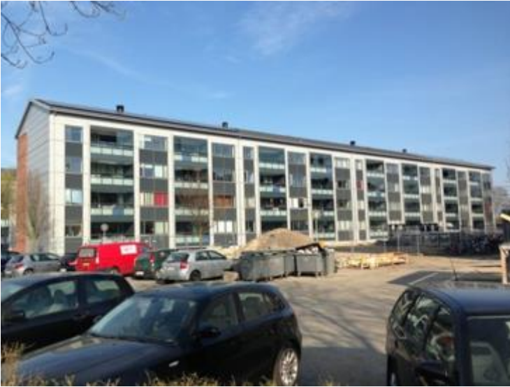
Photo from realisation of large housing retrofit project in Valby at Hornemannsvænge housing estate. 14 kWp PV (100 m 2 ) and 100 m 2 solar thermal is used for each of 6 renovated housing blocks.
