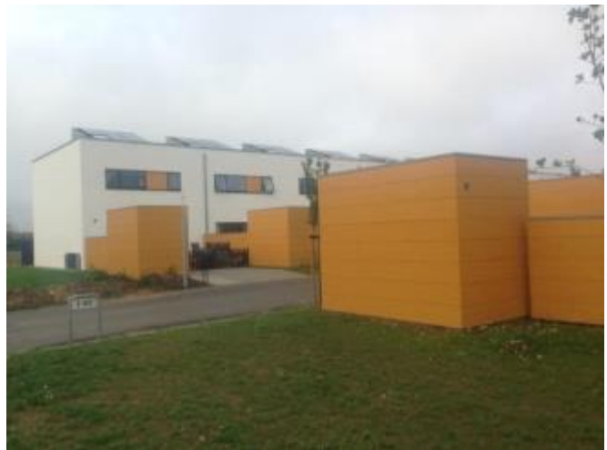
Zero energy housing area with 60 dwellings from 2012 in Tranbjerg Aarhus uses prefabricated Solar Prism systems from Danfoss / VELUX with built in heat pump, HRV system, PV panels and VELUX roof windows.
