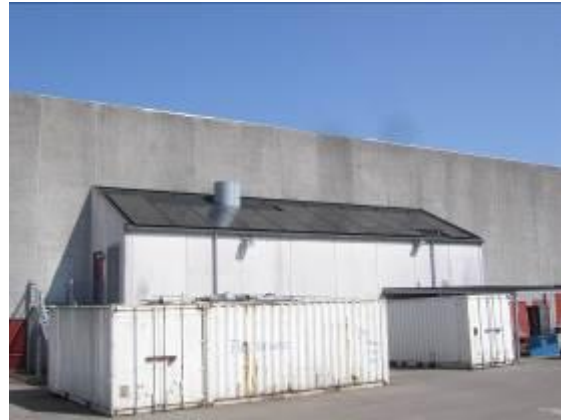
Picture of one of the neighbour buildings with photovoltaic.
