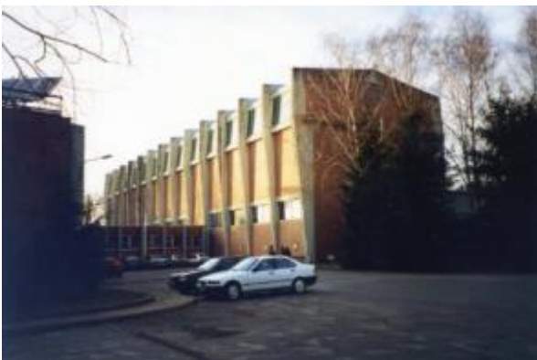
Solar research building at JRC Ispra before renovation
