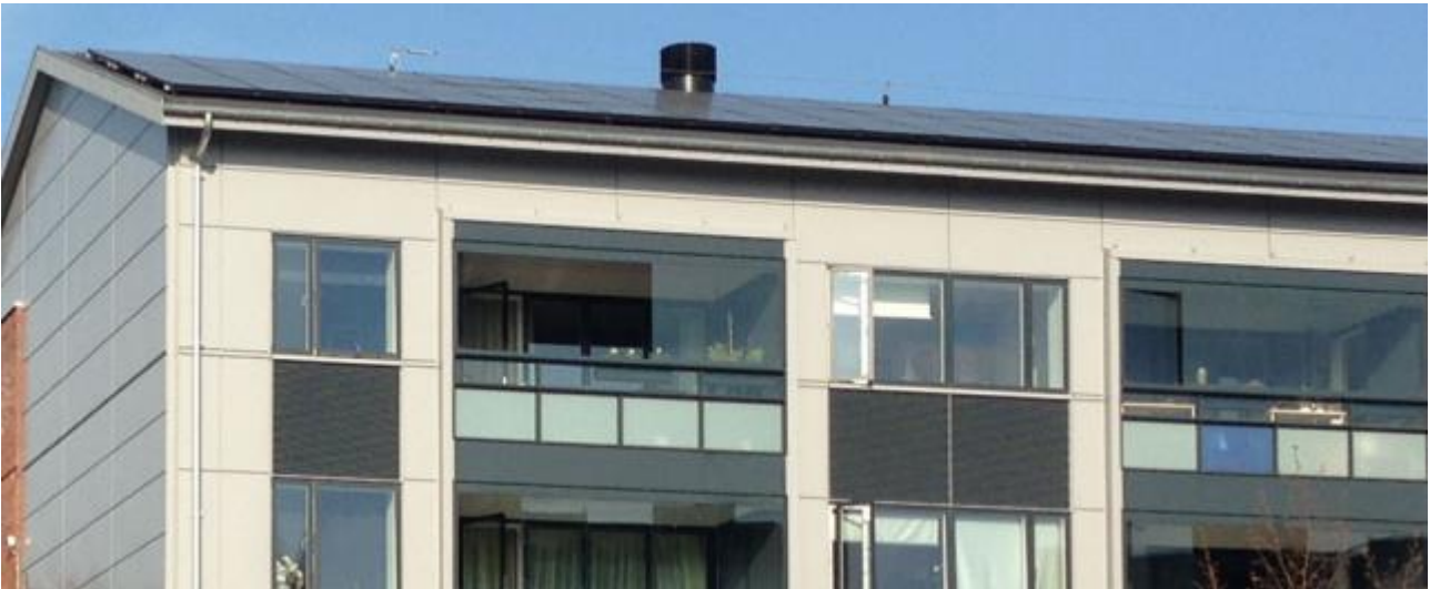
Close up photo of the PV installation on a new sloping roof at the Hornemannsvænge housing estate.
