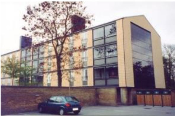
PV integration for an east / west oriented housing block in Skovlunde near Copenhagen based on architectural competition. PV here matched electricity use for ventilation.
