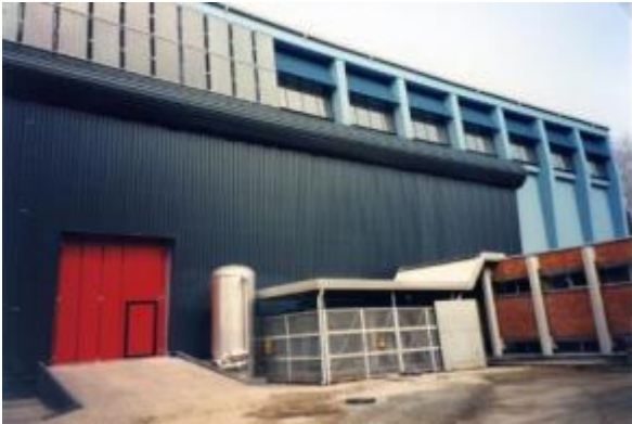
Solar research building renovated with Canadian Solar Wall preheating ventilation air
