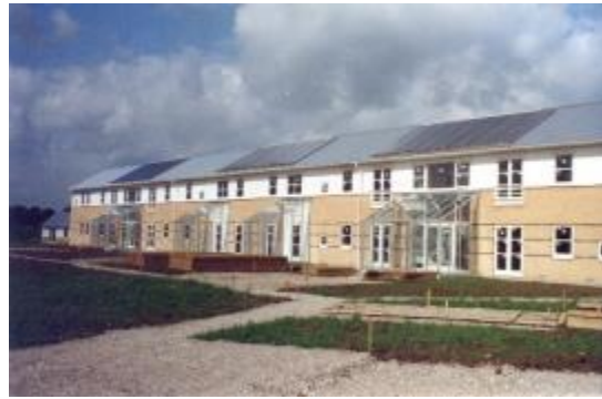
Steel roofs and solar thermal collectors at "Skotteparken"
