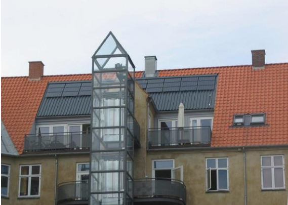
Combined Solar Roof and PV at Frederiksberg
