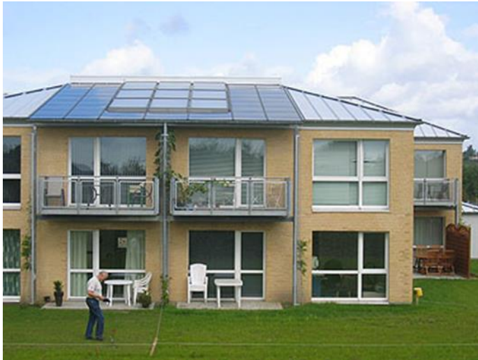
50 m 2 PV-modules in Rønnebækhave II is mounted in the roof facing south in connection to a solar collector area of 28 m 2 . Photo: Peder Vejsig Pedersen
