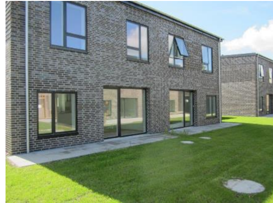
Large window areas towards north will not give problems with overheating and secures good daylight.
