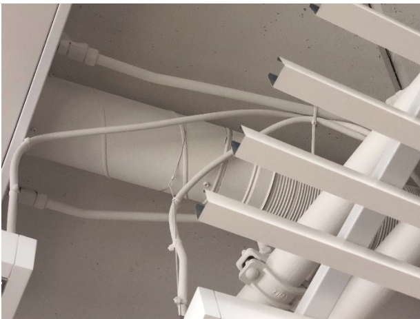
Connection pipes without insulation
