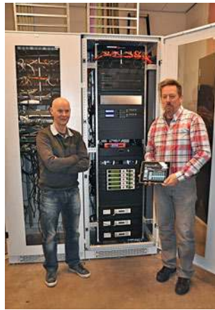
Herman and Arjan. Specialists from B&R Design delivered a complete cabinet with AV equipment and control system Foxtrot (3 pieces at the bottom of the cabinet), which controls the hotel floor with fifteen congress halls.
