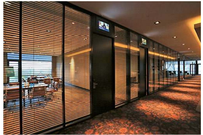
Six separate lounges in a row facing the corridor have glass walls with built-in blinds. They are individually controlled from the control panel in each room.
