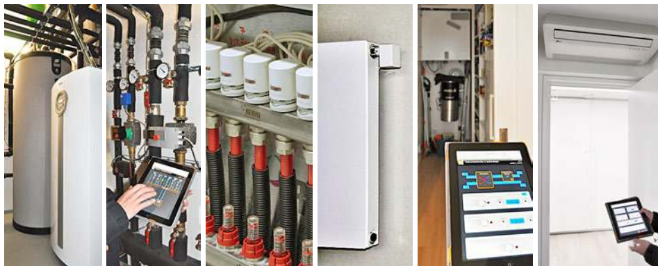
The climate in the house and in every room is controlled by Foxtrot. Starting with the heat pump, the individual heating branches, underfloor heating, radiators, heat recovery ventilation and air conditioning units in every room. Everything is visualized on the tablet.
