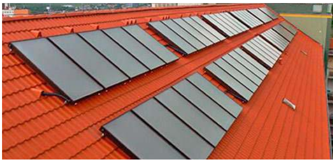
60m2 of SunTime solar panels on an apartment building in Most.
