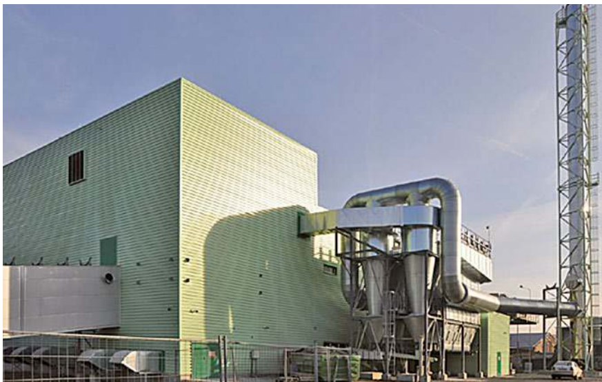
In BIOENERGO COMPLEX in Kolin, Czech Republic, is used system Foxtrot for control of biomass combustion boiler for 6MW generator.
