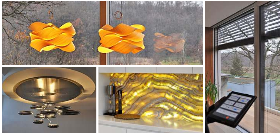
Lutron system controls blinds and window rollers as well as lighting units made by Artemide or backlighting of the onyx kitchen wall. Control pages with graphics shown on a tablet running Elpramo graphics.
