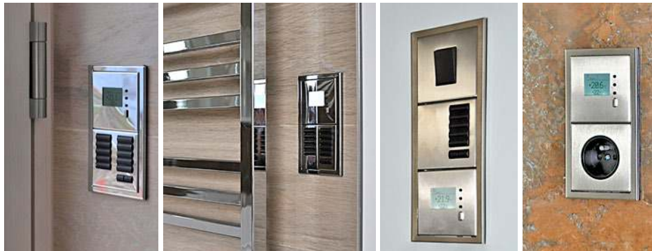
Wall switches with a combination of thermostats C-RC-0003R-Lutron on CIB equipped with multiple press buttons, which are Lutron's specialty – supplied by KD Electronics – and a traditional switch or wall outlet.
