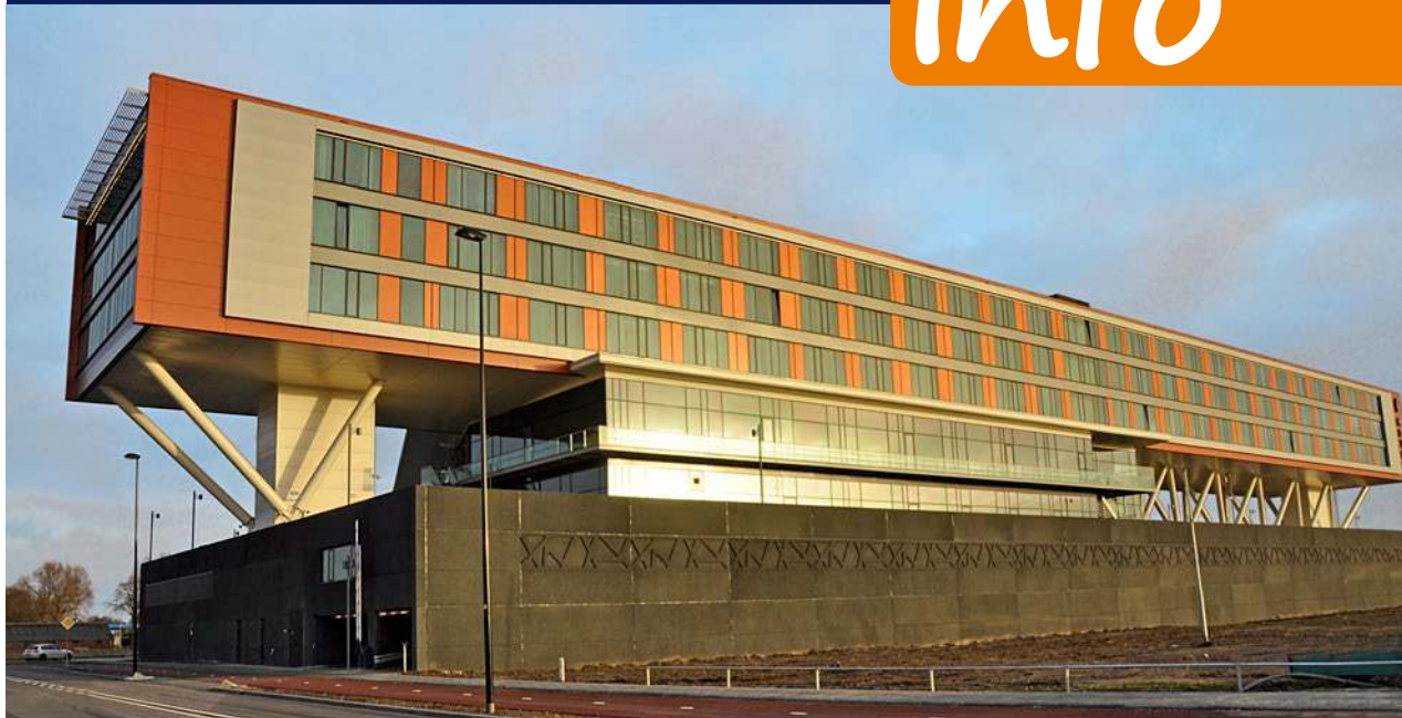
Congress floor of the newest Van Der Valk hotel in Veenendaal, the Netherlands, where one of the latest applications supplied by Tecomat Foxtrot was installed.
