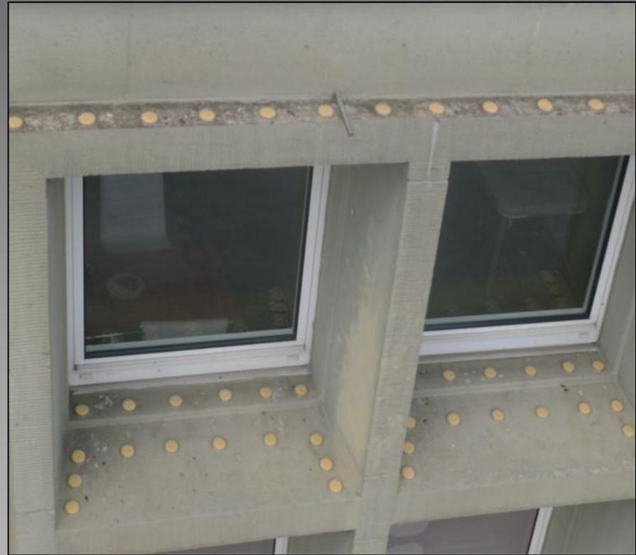
Being a listed building, the local heritage officer would not agree to the use of spikes, wires or nets, while the client wanted a permanent, unobtrusive solution. The building was cleaned of droppings, and 小島 *Bird Free* was installed.
