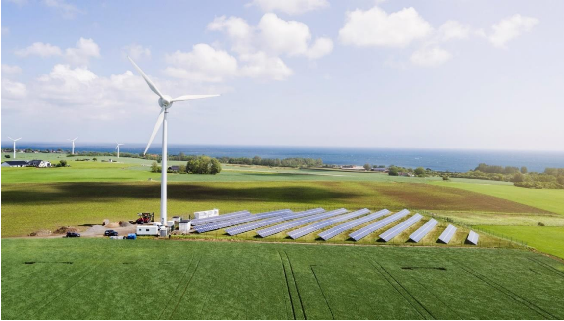
Figure 3: The Simris energy system.
