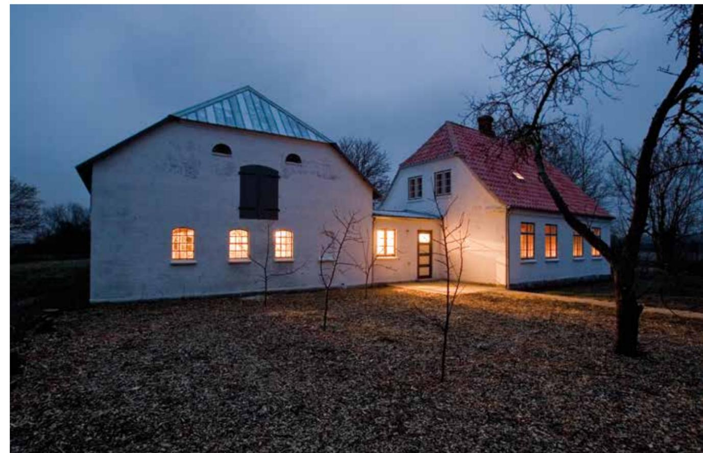
The roof of the farmhouse was finished with new cement wing tiles with the same profile as the original. The original plan was to reuse the old tiles as far as possible and purchase recycled tiles if necessary, but during demolition it became apparent that the tiles were not suitable to be cleaned and relaid. Had it been possible, relaying the roof with only recycled tiles would have saved almost 4.2 kg CO<sub>2</sub> per m<sup>2</sup>.
