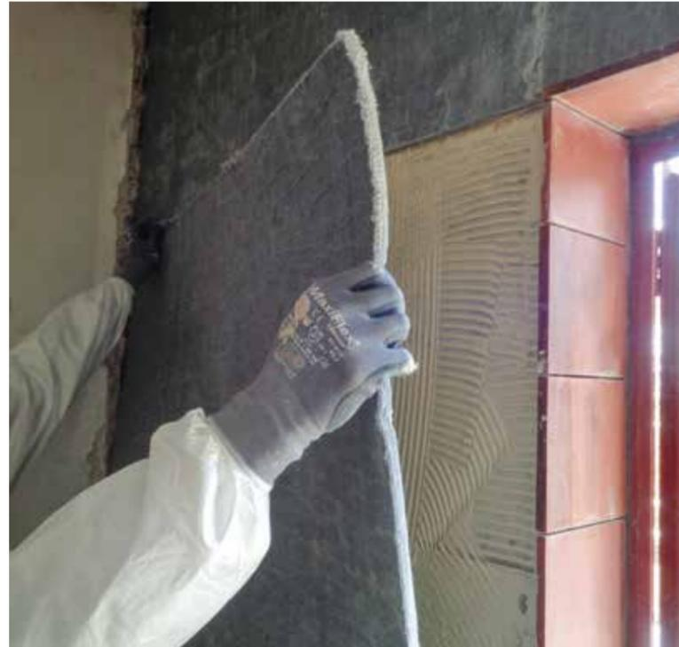
← Fixing aerogel insulation sheets to the walls in Poul Henningsen's house.
