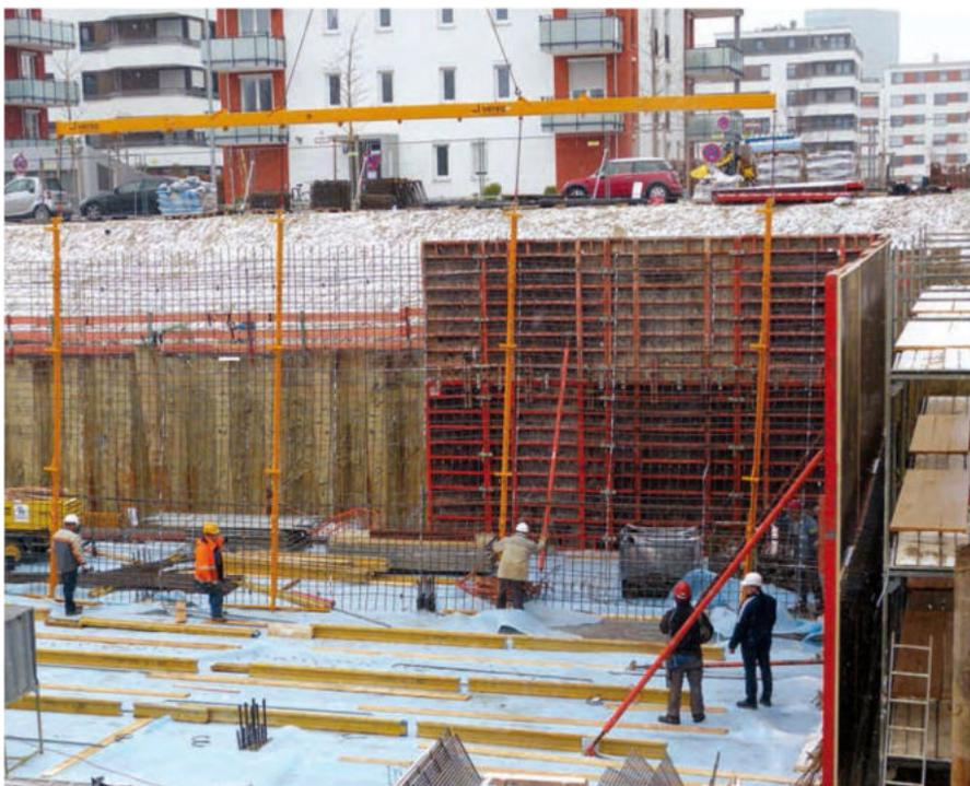
Thanks to the new VRTEC lifting system, BAMTEC reinforcement can be installed rapidly and safely in walls.
