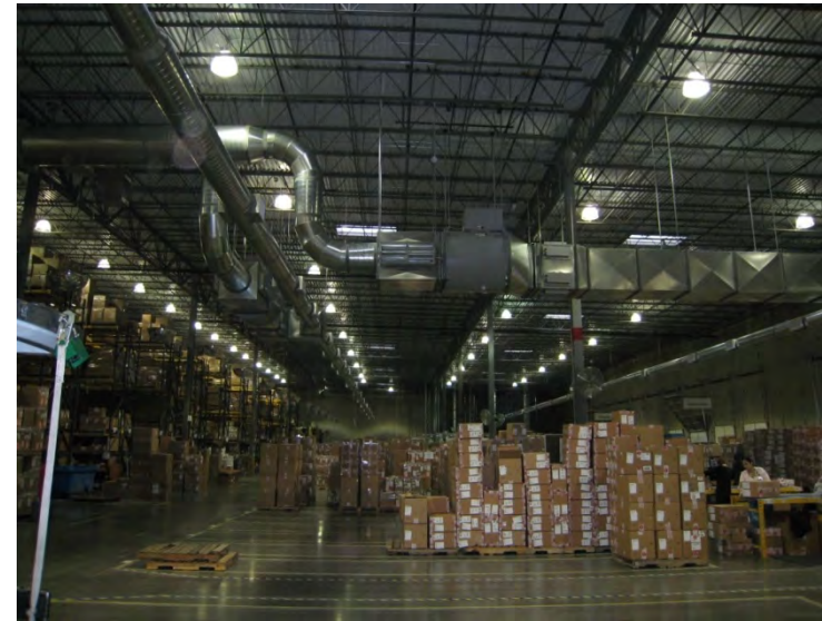
Crocs Distribution Center, Denver, CO, USA Particle and gas elimination in 27,000 m 2
