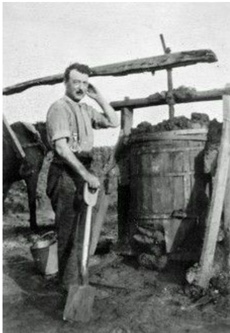
Fig. 2: A great photo of the horse-powered wooden 'Pug Mill', a coopered cylinder that is fed at the top with freshly dug brick making clay. As the horse, clearly seen in Fig. 3, walks
