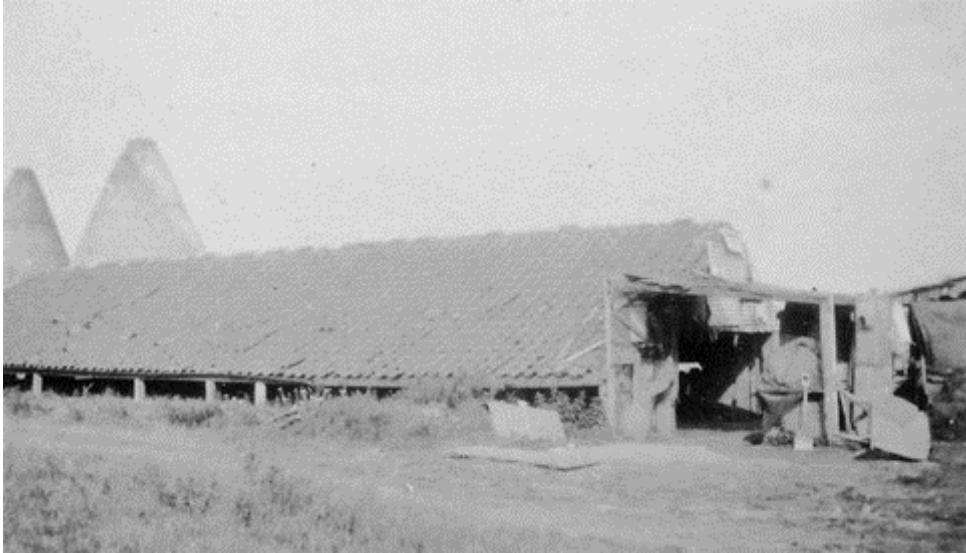
Fig. 1: Setting the scene or this could be the final picture? On the right is a ramshackle shelter where the bricks were moulded by hand. Outside the shelter is a wooden wheelbarrow and spade undoubtedly used for bringing the clay to brick makers. The long, low, pantiled building is the 'Brick Drying Shed' where nearly dry 'green' bricks from a 'hack' may have been herringbone stacked to remove remaining moisture before firing. Any residual moisture in the bricks during firing could cause them to blow apart. On the left may be seen the cones of two brick kilns for firing the bricks. The latter may be a clue as to the brickyard's location.
