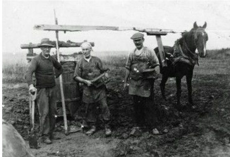
Fig. 3: With the 'Pug Mill' situated near the brick moulding area, the whole arrangement can be clearly seen; including the horse hitched to a somewhat dodgy looking sweep arm. The duty of the man on the left is to feed the pug mill with clay. The horse almost certainly works automatically to voice commands. The two men centre and right are brickmakers as defined by the wooden brick moulds that they hold in their hands.
