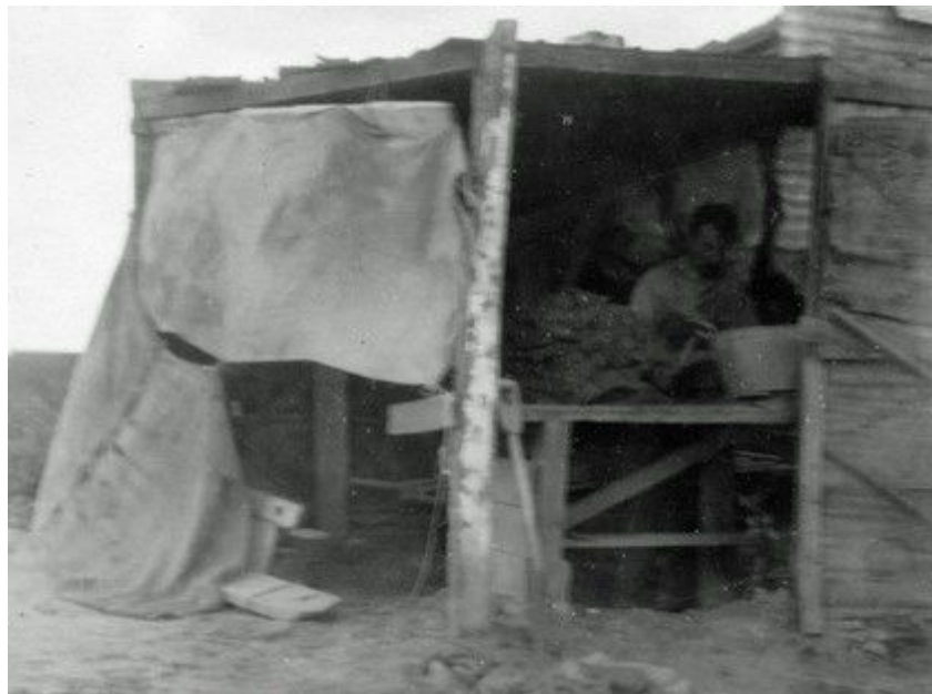
Fig. 4: This vernacular, ramshackle hovel is the brick making shelter. The brick maker is stood behind his bench that is heaped with clay from which he will cut enough to, with a well-aimed throw, fill a brick mould before striking it level. The bucket in front of him probably held sand with which he would sand the moulds before filling them.
