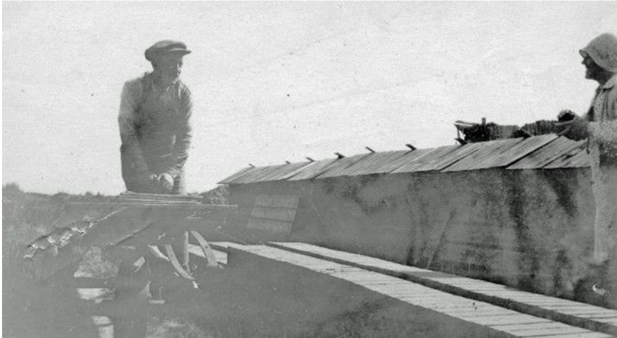
Fig. 7: Although not the clearest photo, the brickmaker is stood with the hack barrow beside a new hack that he is building. Behind the ongoing hack is a completed one with weather protection hack boards sat on top and to the side. After initial drying in the hack the bricks might have been taken to the long, low brick drying shed ( Fig. 1 ) where now dry enough to be stacked in such as herringbone pattern with ventilation breaks, they would remain to finish drying until deemed ready to be fired in the kilns. © Bob Powell, Kingussie
