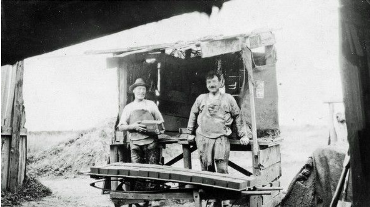
Fig. 5: In this better view of the brickmaking shelter the man on the left is holding a brick mould. The single wheel barrow in front of the men is a 'Hack Barrow' onto which are loaded the newly moulded bricks that have been turned out on to individual boards that are slightly larger than the mould. From here the wet bricks are barrowed to a 'Hack' where stacked, they begin their air drying process in advance of firing.
