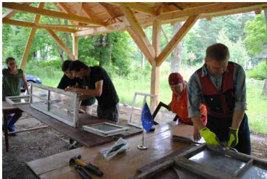
Photo 2 Restoring old windows
