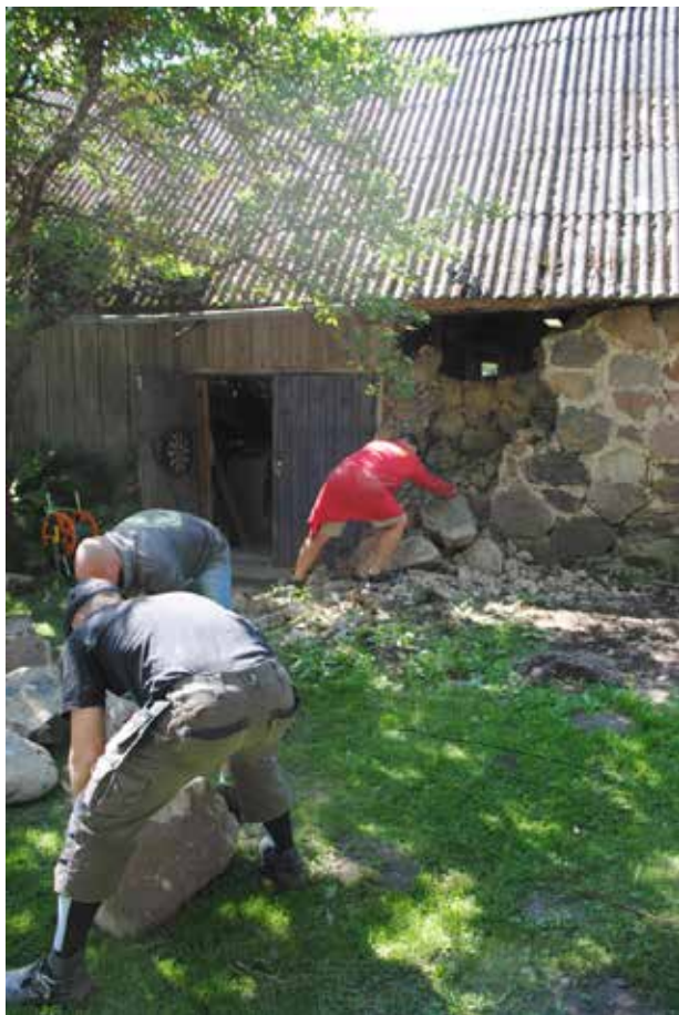
Photo 1 Restoring granite walls
