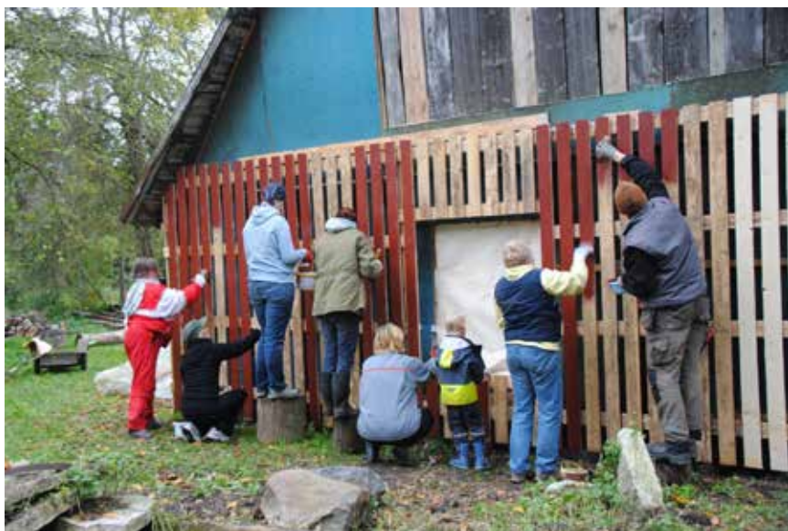
Photo 3 Traditional paints 2012 in Rapla County
