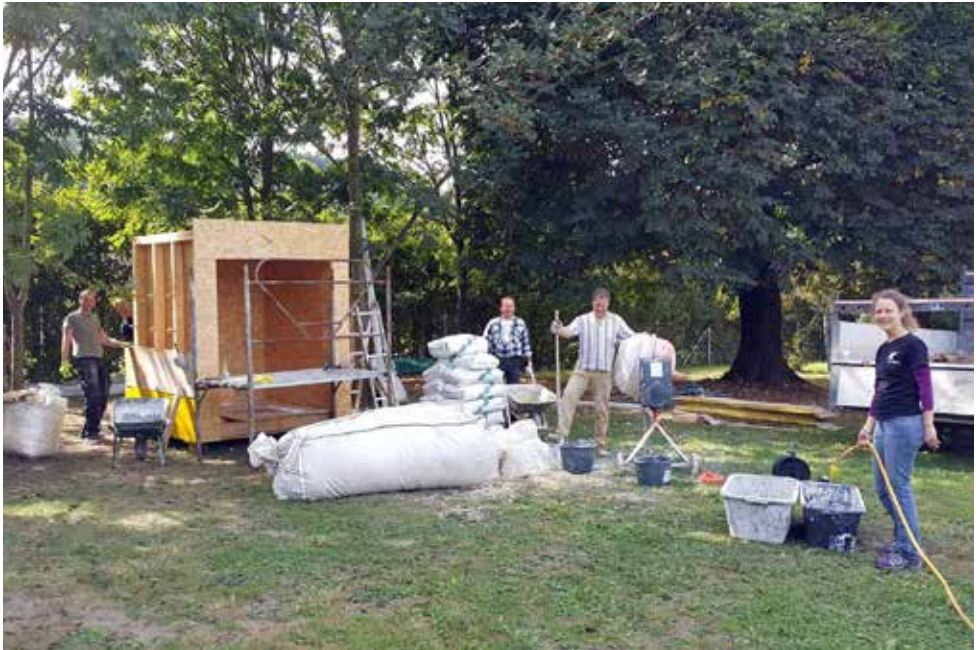
Photo 6 Building a sauna from hempcerete
