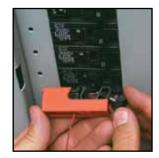
2. Attach the lockout device to the breaker and snap into locked position.
