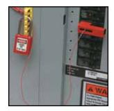
3. Pass plastic key through lock rail and attach lock, preventing key from sliding down cable and opening lockout device.
