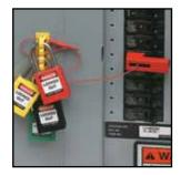
For group lockouts, run key through multiple loops in lock rail and apply locks. No hasps required!
