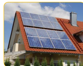
Solar roof project
