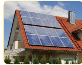
Solar roof project
