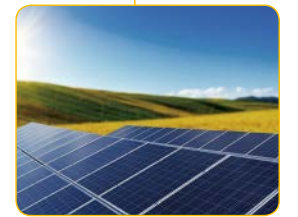
Solar power station
