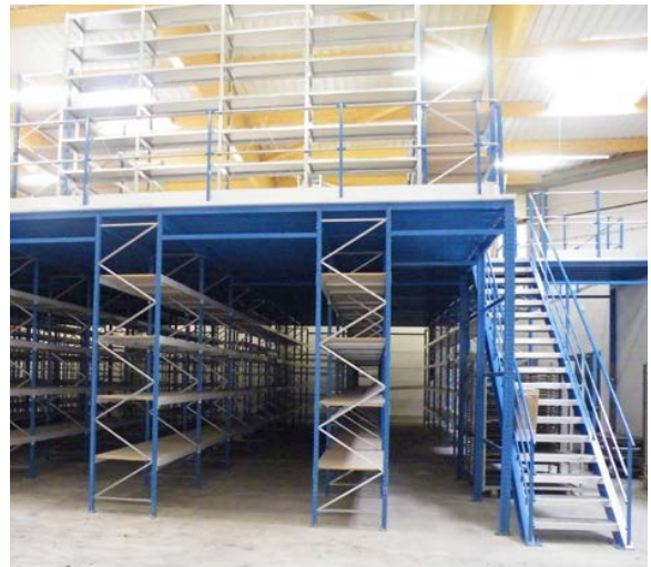
Mezzanine over Epsivol shelving.
