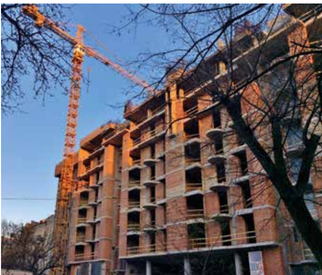
Fig. 2: The new construction at Gonchara str., 17-23.
