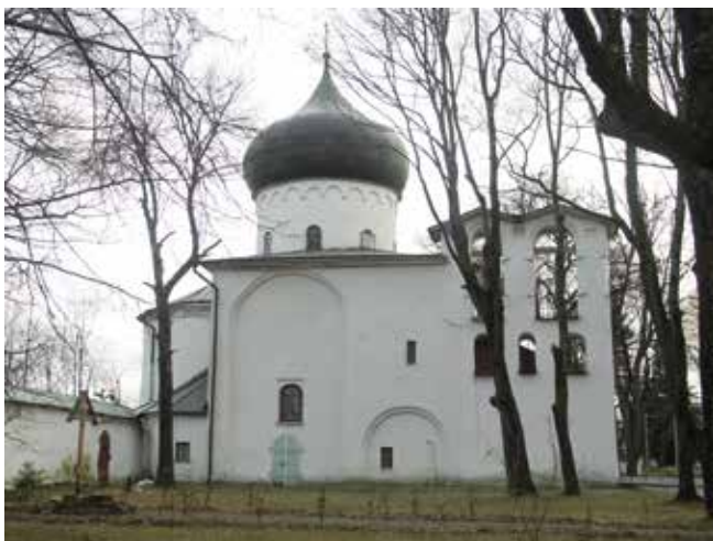
Fig. 1: The Transfiguration Cathedral of the Mirozh Monastery.
