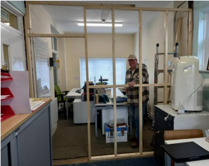
We built a dividing wall to separate a large office into two smaller work areas.
