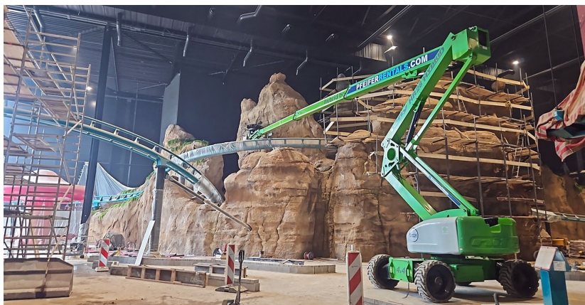
Bommelwereld under construction
