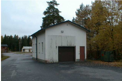
Explosives area LV3
