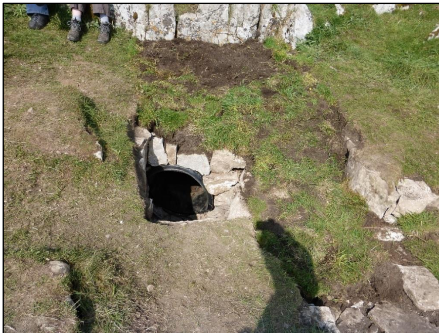
The finished entrance to Hags Brow Cave.
