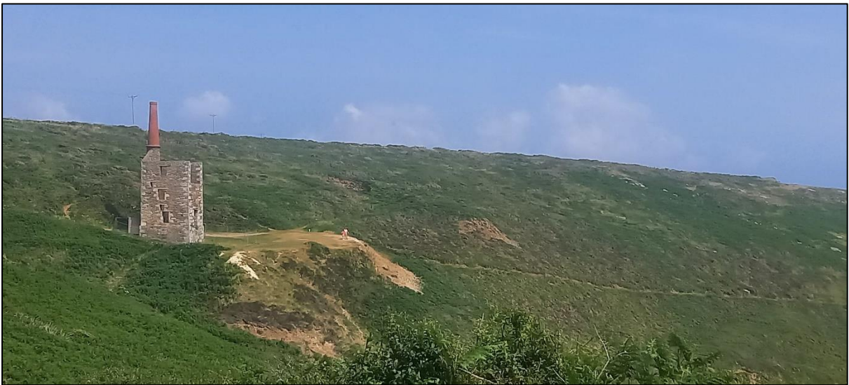
Wheal Prosper (built 1860) at Rinsey, southwest facing aspect, 13/06/23
