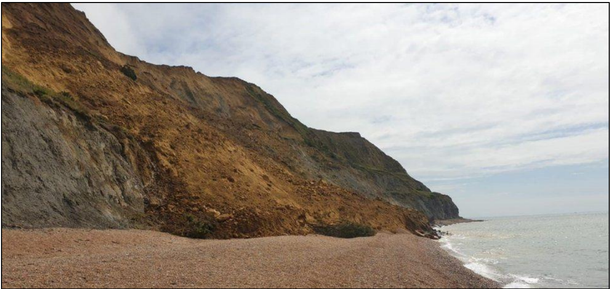
IMAGE SOURCE, DORSET COUNCIL A section of cliff has collapsed cutting off a stretch of beach on the Jurassic Coast.
