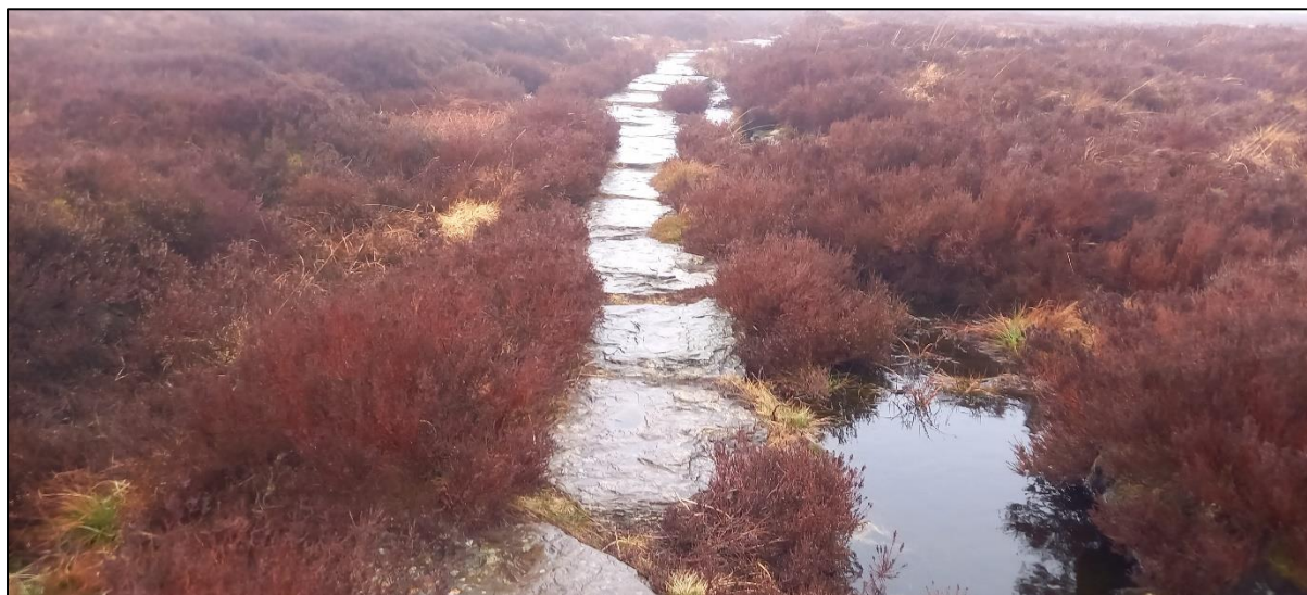
Flagstone path over peat hag, Hatterrall Ridge
