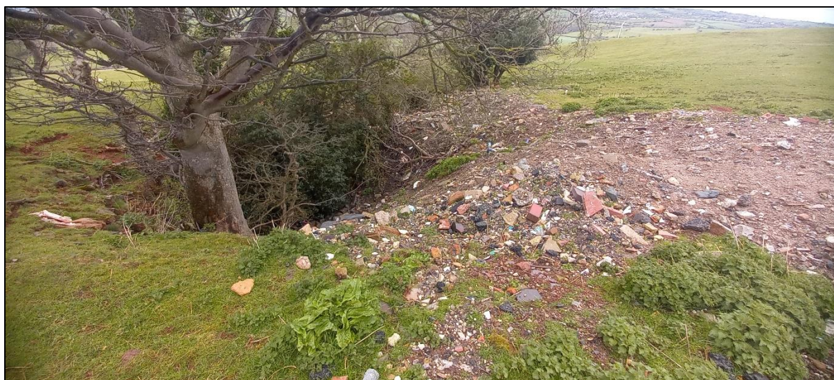
Naturally occurring karstic feature partially backfilled with demolition rubble and other rubbish!
