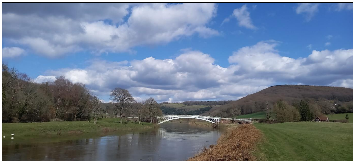
Bigsweir Bridge over the River Wye
