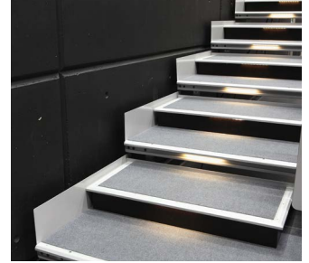
Kick plates - To guard the operational clearance where an aisle is adjacent to a wall.
