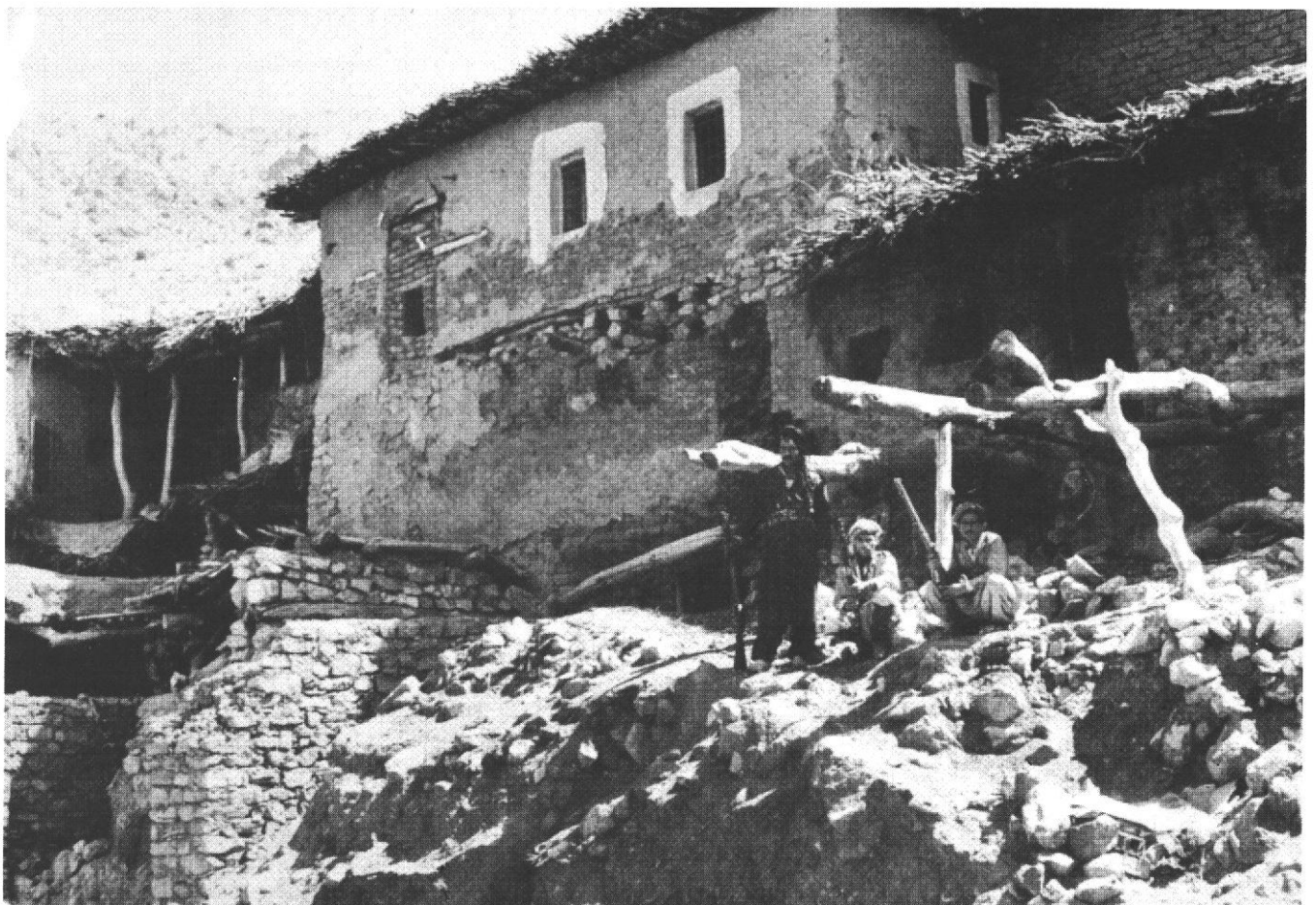
A bomb-damaged house at Galala.
