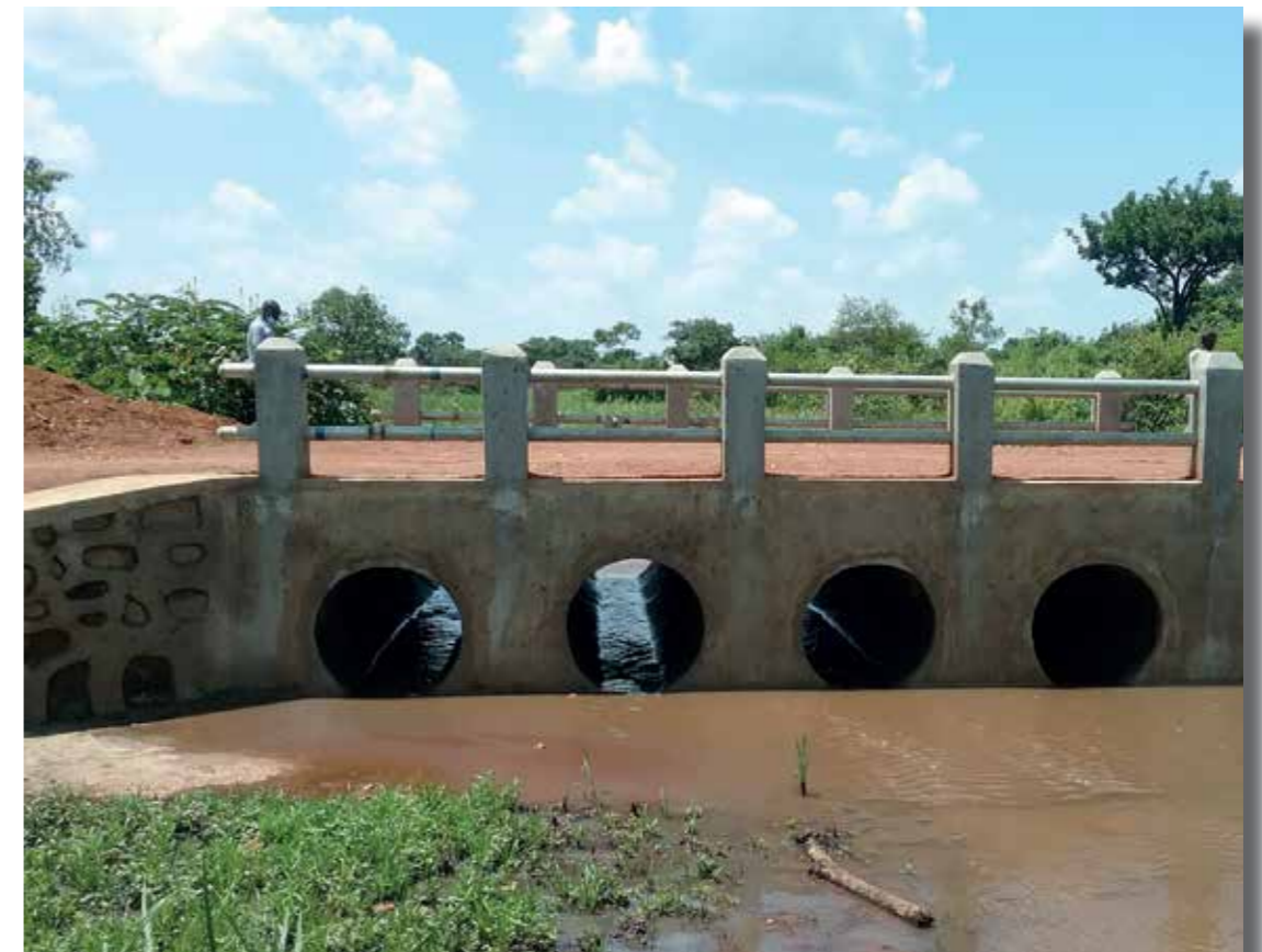
Vented Drift along Manibe-Ewadri-Kasikasi road - Arua District
