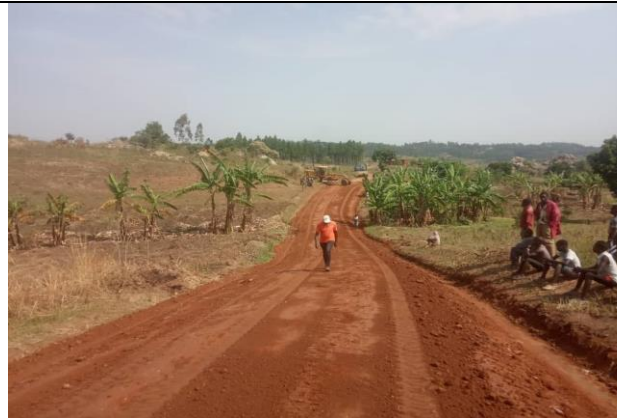
Compaction of gravels on Goli to Omunda GR4W, Nebbi district
