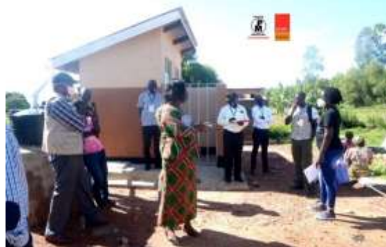
VIP latrine constructed at Komite parish market
