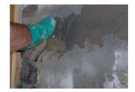
The material is based on a blend of cement, graded aggregates, special fillers and chemical additives which control the rate of set and minimise the risk of thermal cracking. Renderoc Plug provides an initial set time of approximately one minute.
