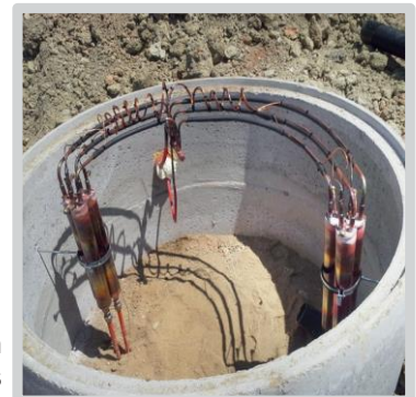
3. Well with CO 2 -Probes
