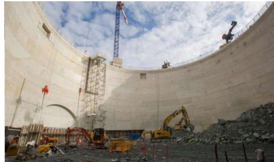
Production of Diaphragm Walls
