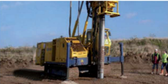
Project: Resin stabilised permeable vibrated stone columns
