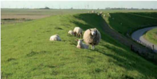
Project: Geological solidification as well as sealing to damaged dams and dykes.
