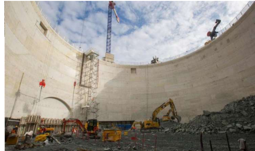
Production of Diaphragm Walls
