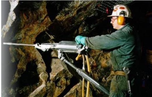
1) Drill Bolt Hole
