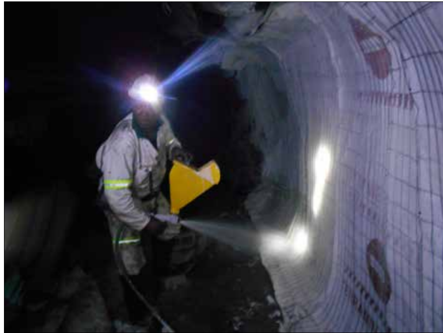
Handling of ROKTAK® Gun and Hopper underground
