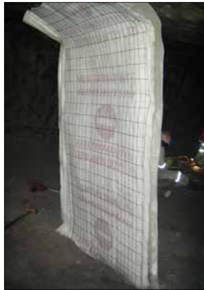
VENTMESH® Lite PP (Polypropylene) Installation
