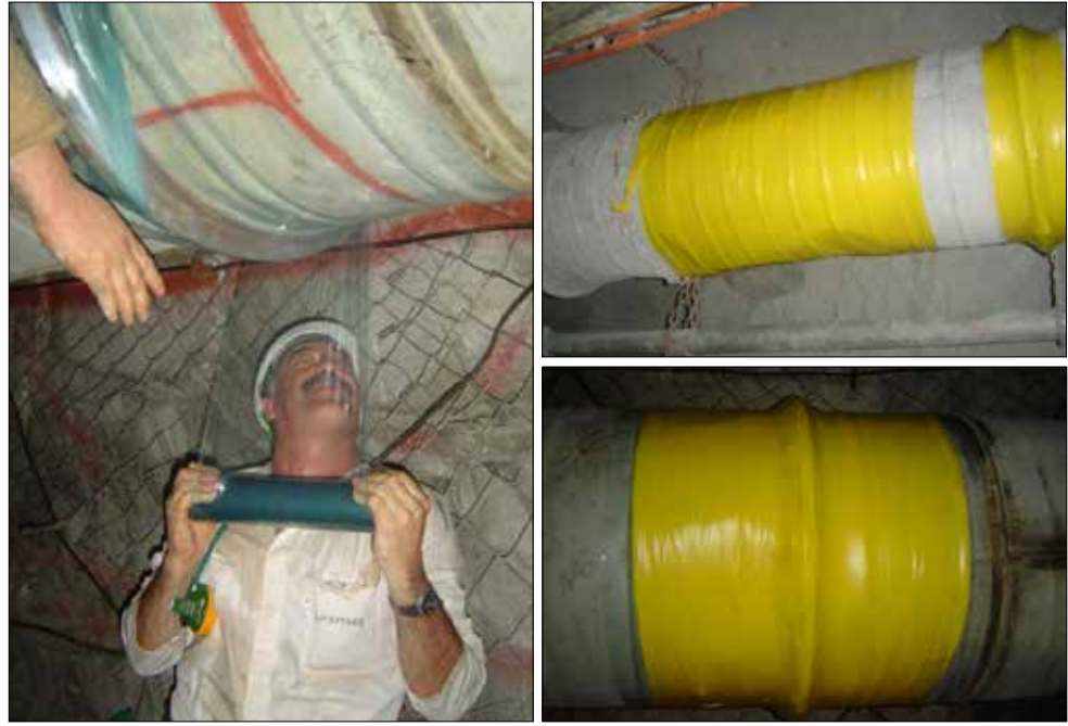
SEALADUCT® 80 being applied to a leaking column
