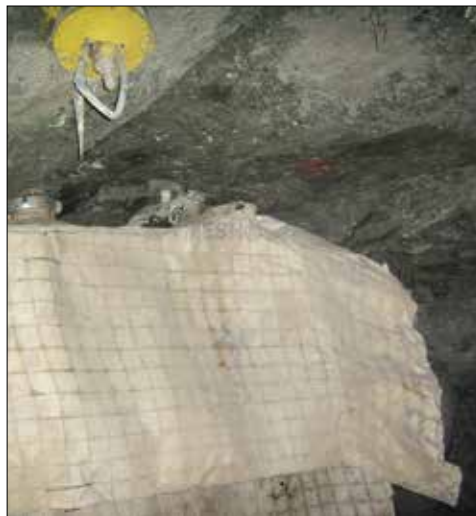
VENTMESH® Lite Combo installed in a Vent Seal
