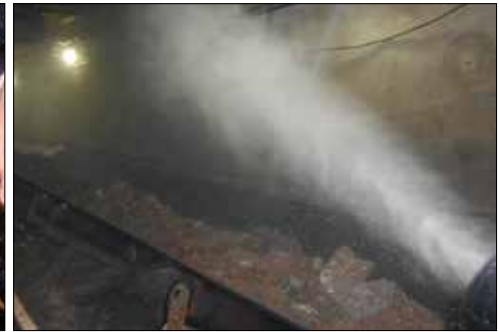
Adjusting TERRABLAST® underground
