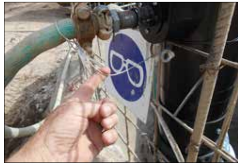
Airmover Installed with Safety Sling (attached to air supply)
