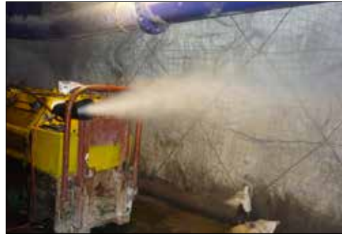
TERRABLAST® Application Underground
