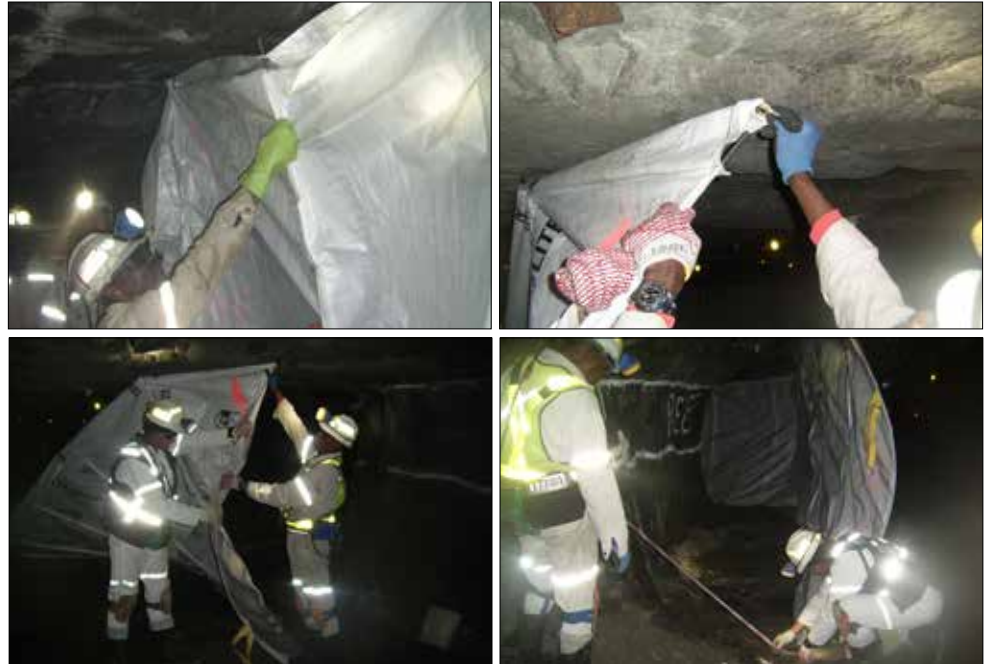
Underground Installation of VENTICORSET™
