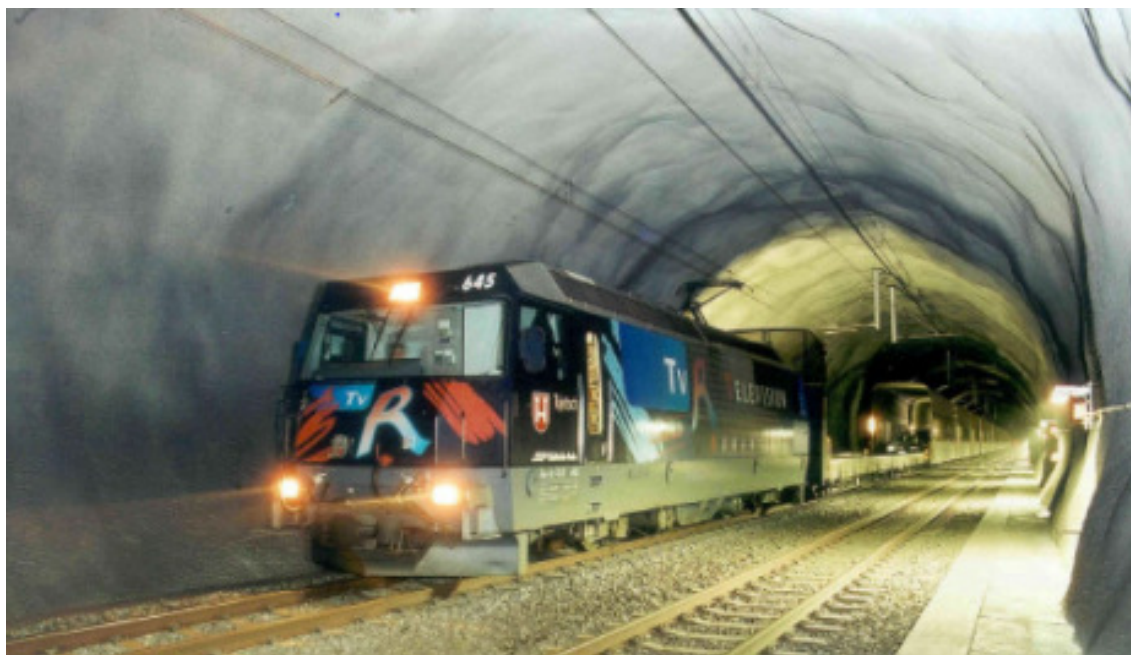
Figure 9: The Vereina tunnel in operation
