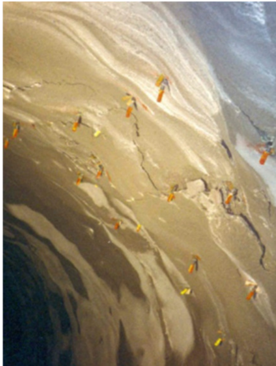
Figure 8: Squeezing ground supported by GFRP bolts and sprayed concrete
