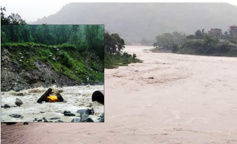
Excavators being swept away by the flood in the Super Madi Hydropower Project in Kaski.
