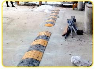
TOTAL FILLING STATION, MFAMOSING CALABAR
