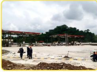
TOTAL FILLING STATION, MFAMOSING CALABAR
