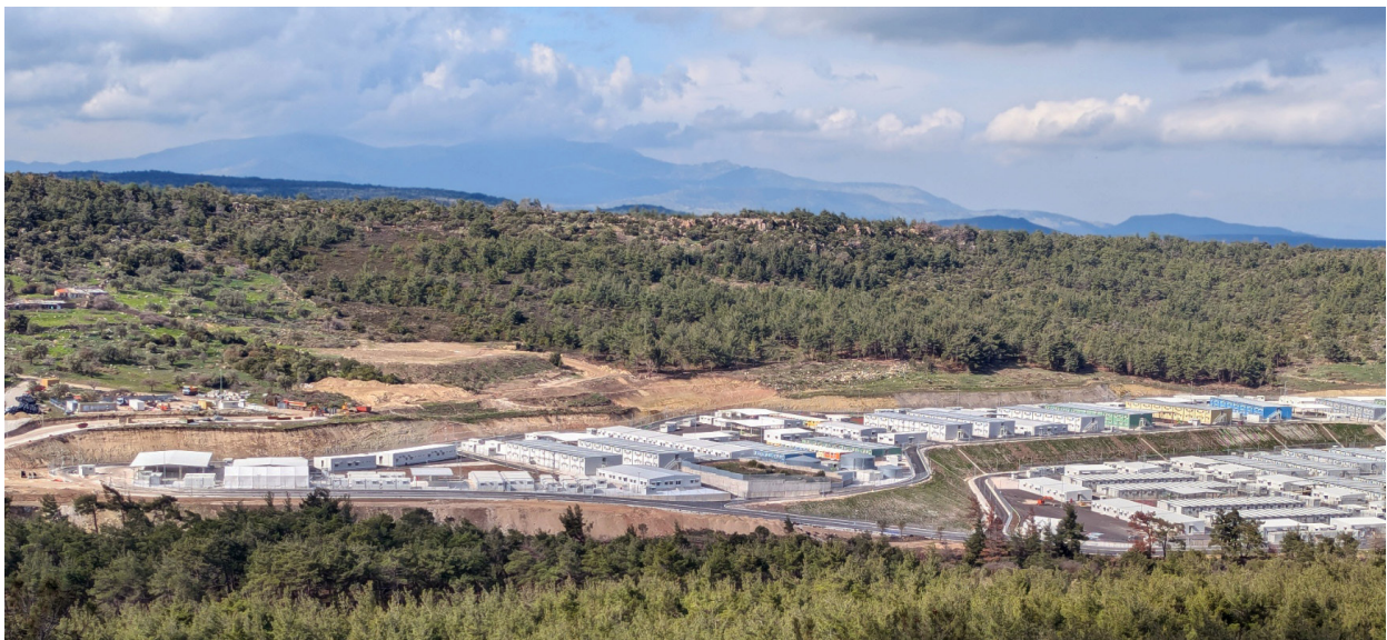
Photo: Vastria construction site as of February 2025. Source: Anonymous
