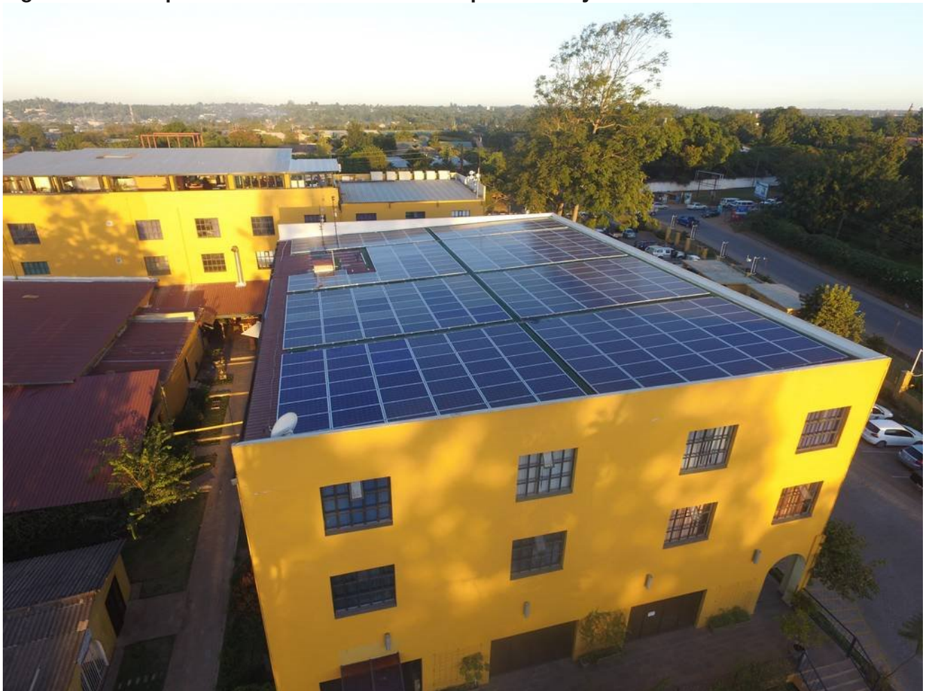
Figure 16: Aerial photo of Foxdale Court's rooftop solar array
