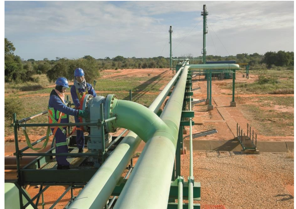
Image: Engineers work on Rompco gas pipeline, Mozambique
