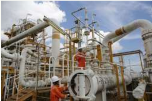
Petroleum Pipeline Inspection And Repair Process
