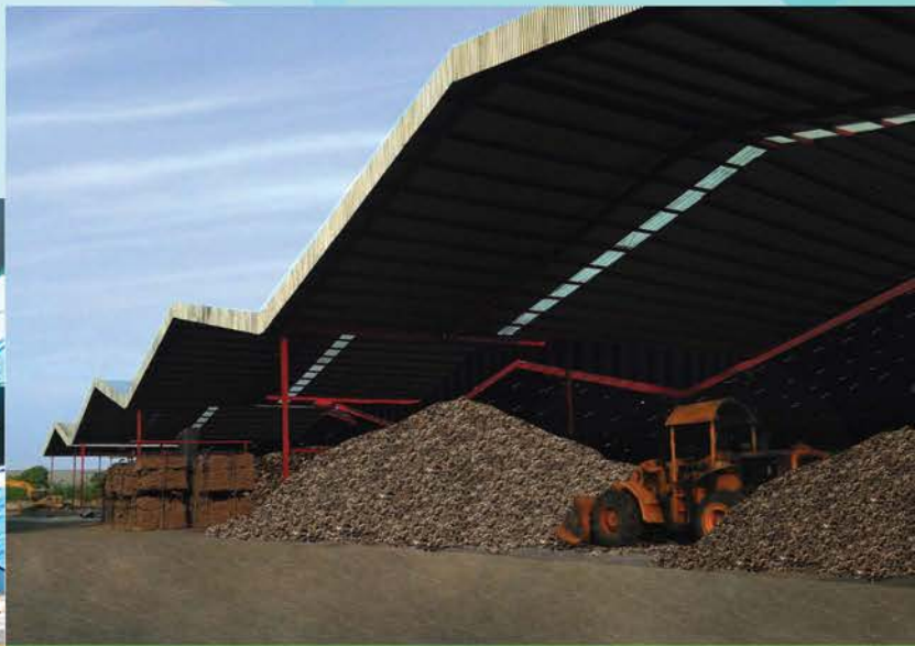
NEW EXPANSION FACTORY FOR AGING CRUMB DRC AND BLENDING SYSTEM
