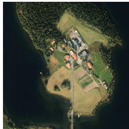
The main area of the prison is located in the centre of the island. Photo: Gule sider
