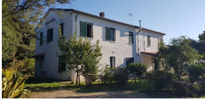
APG Houses Italy
