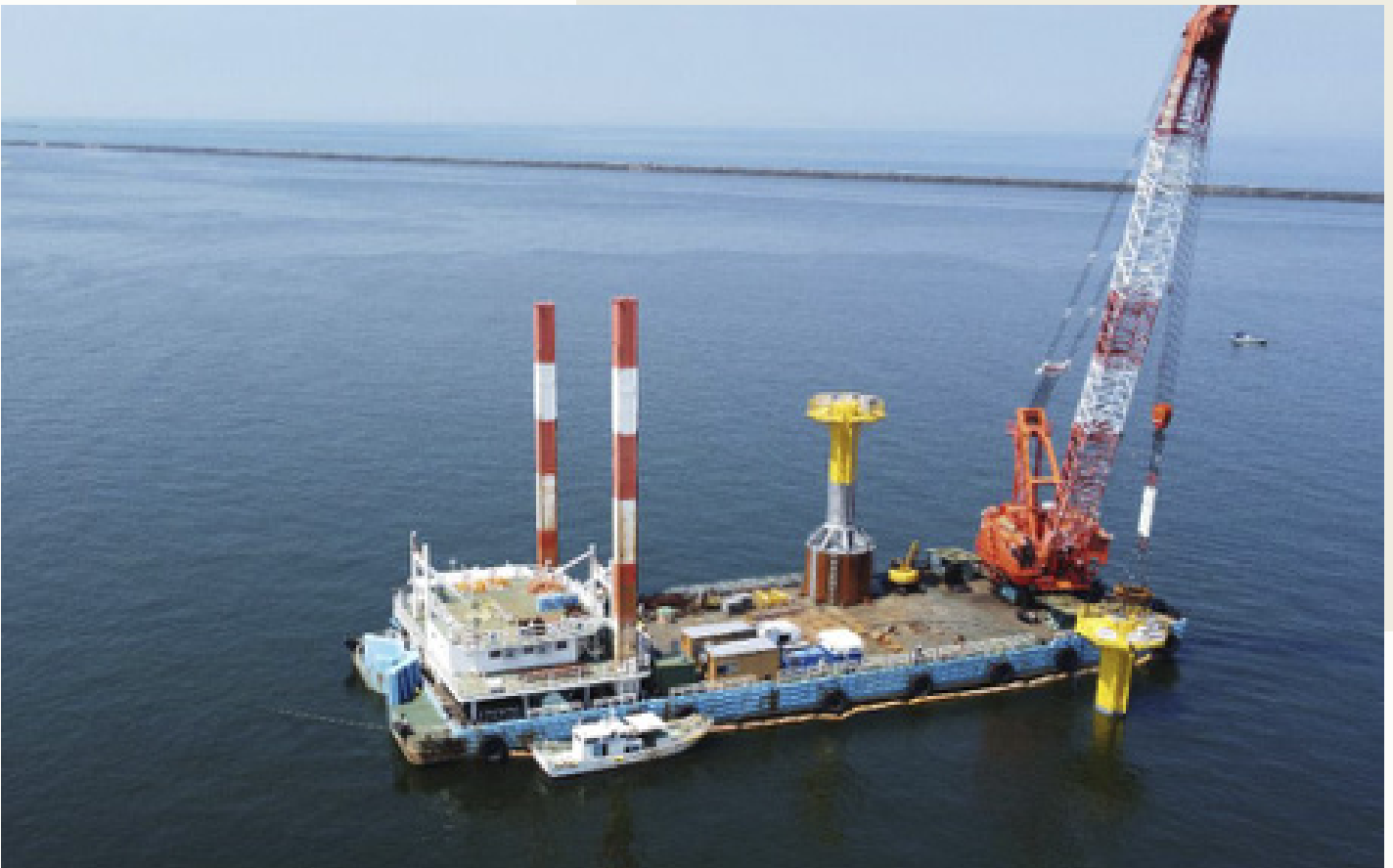
Figure 3: Demonstration of base construction technology for suction buckets in actual sea area.
