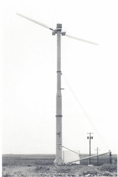
Figure 1. The 80-kW Lagerway wind turbine operated by Dutch Industries Ltd. at Cambridge Bay, Northwest Territories.
