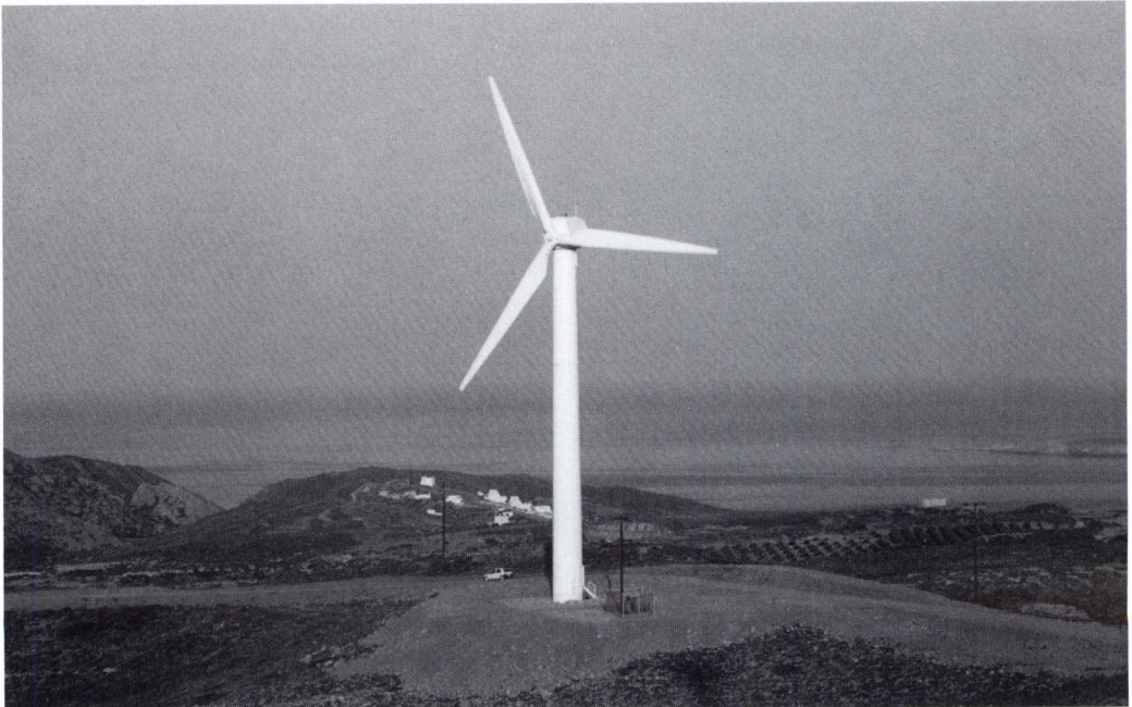
Figure 3. One of the 500-kW wind turbines installed by PPC in Moni Toplou, Crete, in the framework of the Thermie demonstrator program of the EU.
