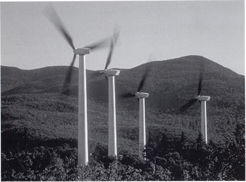
Figure 1. Green Mountain Power 6-MW wind power plant near Searsberg, Vermont. Twelve 550-kW Z-40 wind turbines were installed.
