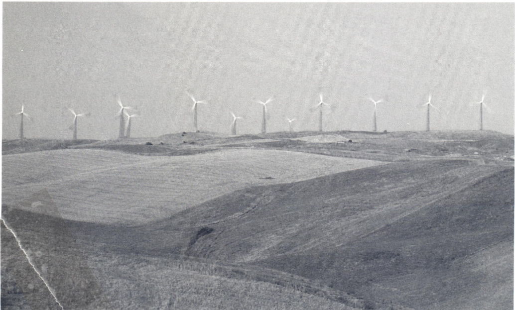
Figure 3. The 7.2-MW wind power plant built by the IVPC Company at Montefalcone Val Fortore (Campania–Southern Italy) with 12 Vestas V42 machines (600-kW rated power).
