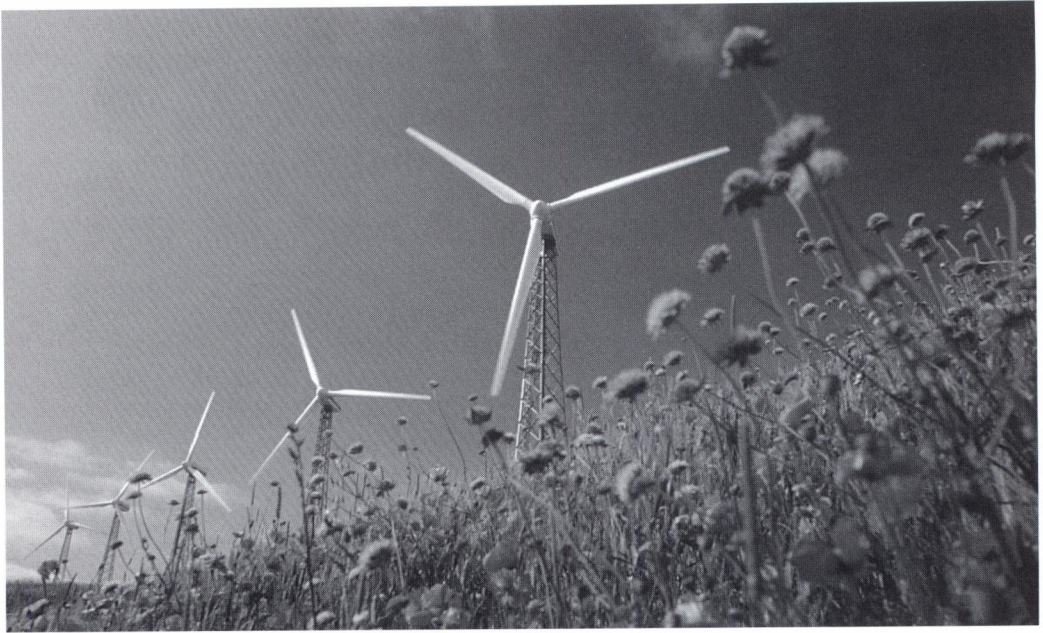
Figure 4. The 3-MW wind power plant set up by IVPC at Alberona (Apulia–Southern Italy) with five Vestas V42 machines.
