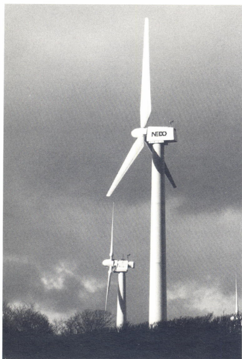
Figure 1. NEDO 500-kW WTGS at Tappi wind power plant.
