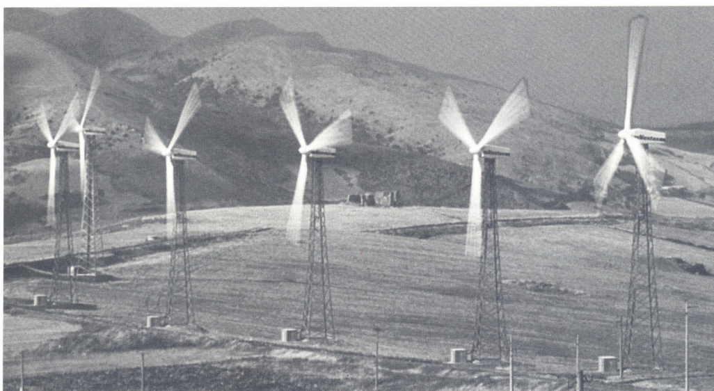
Figure 5. The 3.6 MW wind power plant built by IVPC at Sant' Agata di Puglia (Apulia, Southern Italy) with six Vestas V42 machines.
