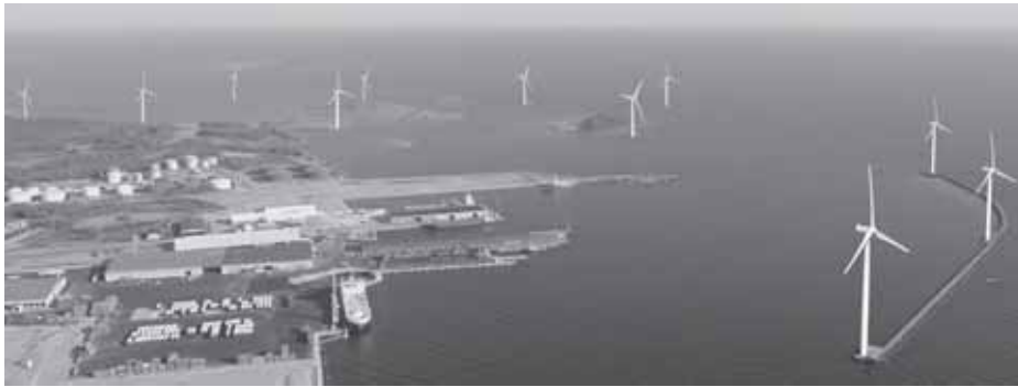
Figure 4 Photo montage of the semi-offshore wind farm in Kemi, where ten 3-MW turbines are to be built in 2007 and 2008. The existing 3-MW power plant can be seen as the left-most turbine (Photo: H. Wallas).
