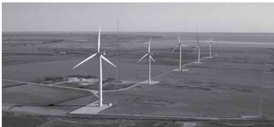
Figure 6 Test site at Hovsore.
