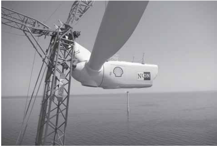
Figure 4 Construction of Offshore Wind farm Egmond aan Zee (OWEZ). Photo G.Pascaud, A2SEA.
