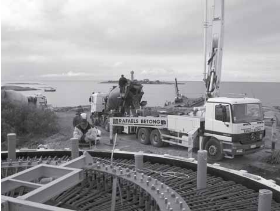
Figure 3 Building the foundations on the cliffs and small islands in Åland archipelago, Båtskäer (Photo: Henrik Lindqvist).
