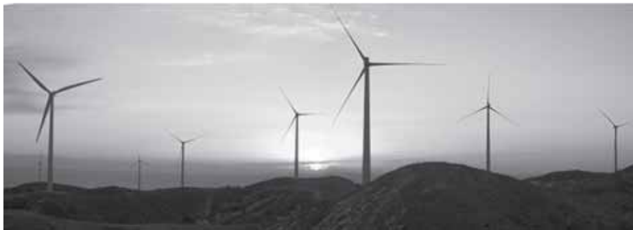
Figure 1 Yongdeok Wind Farm faces the East Sea of Korea; twenty-four units of 1.65-MW NM82 (V82).
