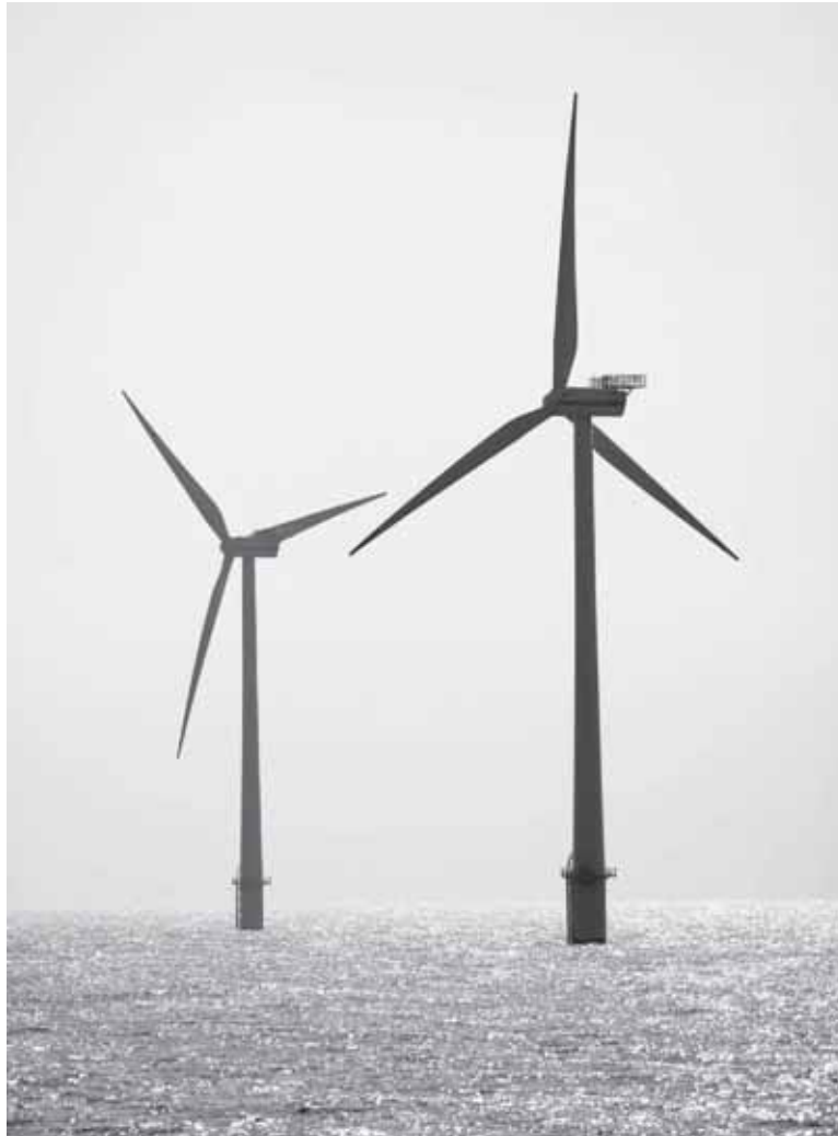
Figure 5 Two of the eighty turbines at the Horns Rev 160-MW offshore wind farm (published with permission of DONG Energy and Vattenfall).
