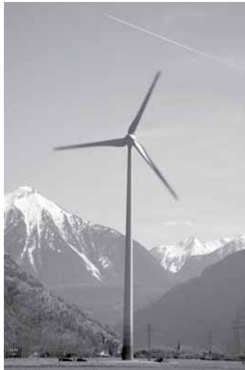
Figure 2 The Enercon E70 in Collonges. The new workhorse for wind energy in Switzerland performs with a capacity factor of 25% and is responsible for 28% of the total energy yield from wind power. Photo by Suisse Eole (Chevalley)
