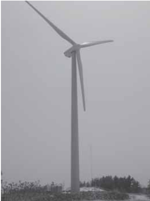
Figure 3 Hanjin's 1.5-MW wind turbine.
