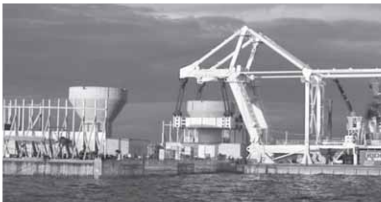
Figure 5 Lifting of foundation at Lillgrund (Photo credit: Hans Blomberg, Vattenfall AB)
