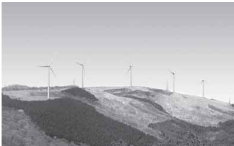
Figure 6 Ichimokusan Wind Farm.
