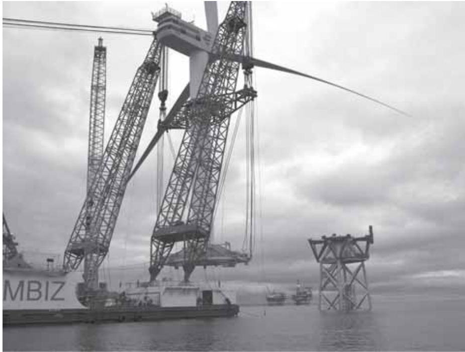
Figure 13. DOWNVIInD: The first of two RE Power 5-MW wind turbines being lifted towards its foundation; the Beatrice platform is visible in the background.
