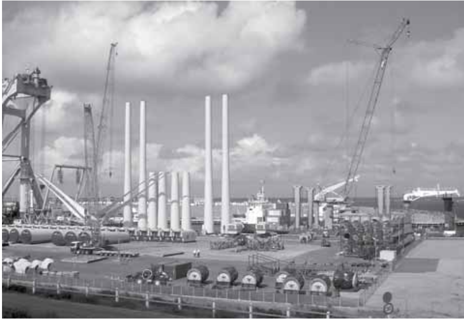
Figure 2 Offshore Wind Farm Egmond aan Zee (OWEZ) construction yard, IJmuiden harbor. Towers, blades, nacelles are shown. Photo J.L. 't Hooft, SenterNovem.
