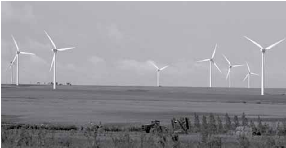
Figure 3 Centennial Wind Farm (150 MW) in Rushlake Creek, Saskatchewan. (Photo Credit: Jimmy Royer 2006)
