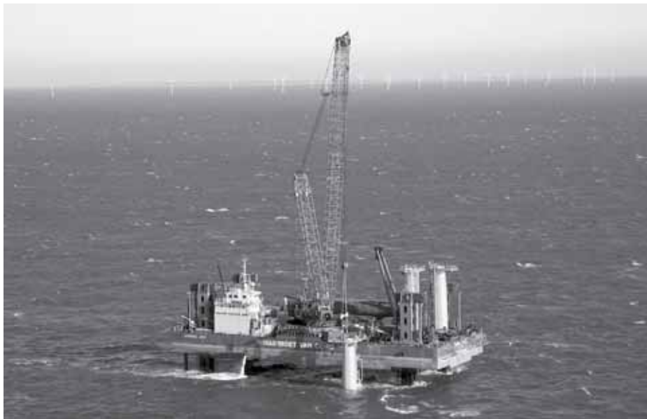
Figure 5 Picture of Jumping Jack placing a transition piece on Q7 monopile. In the background the OWEZ. Photo Mammoet van Oord.
