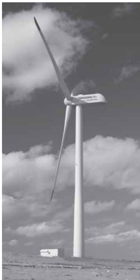
Figure 4 FHI's new 2-MW, downwind-type wind turbine, the SUBARU 80/2.0, installed at Hazaki.
