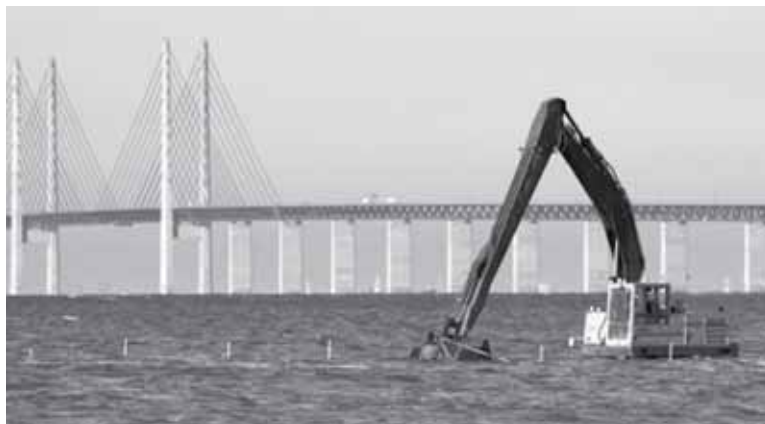
Figure 4 Cable-laying work at Lillgrund (Photo credit: Hans Blomberg, Vattenfall AB)
