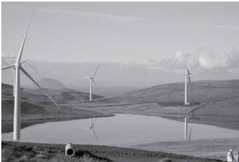
Figure 12: The UK’s largest capacity onshore wind farm, Hadyard Hill, 119.6 MW, located in Barr, South Ayrshire; online in March 2006.
