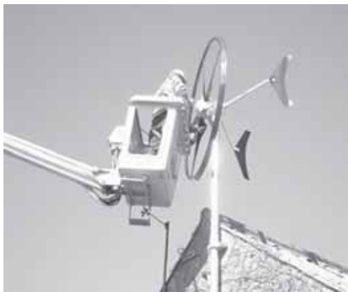
Figure 10 A typical Swift wind turbine during installation (photo courtesy of Renewable Devices Energy Solutions Ltd © 2006).
