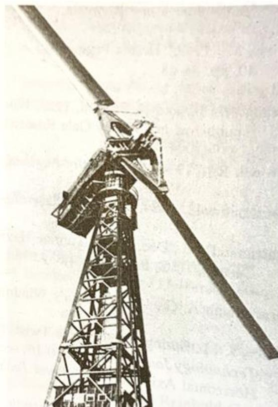
Figure 1 Smith-Putnam 1,250 MW two-bladed downwind turbine.
