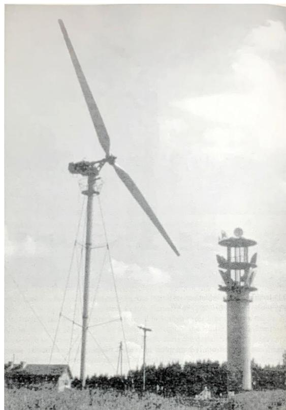
Figure 2 Hutter 100 kW two-bladed downwind turbine.
